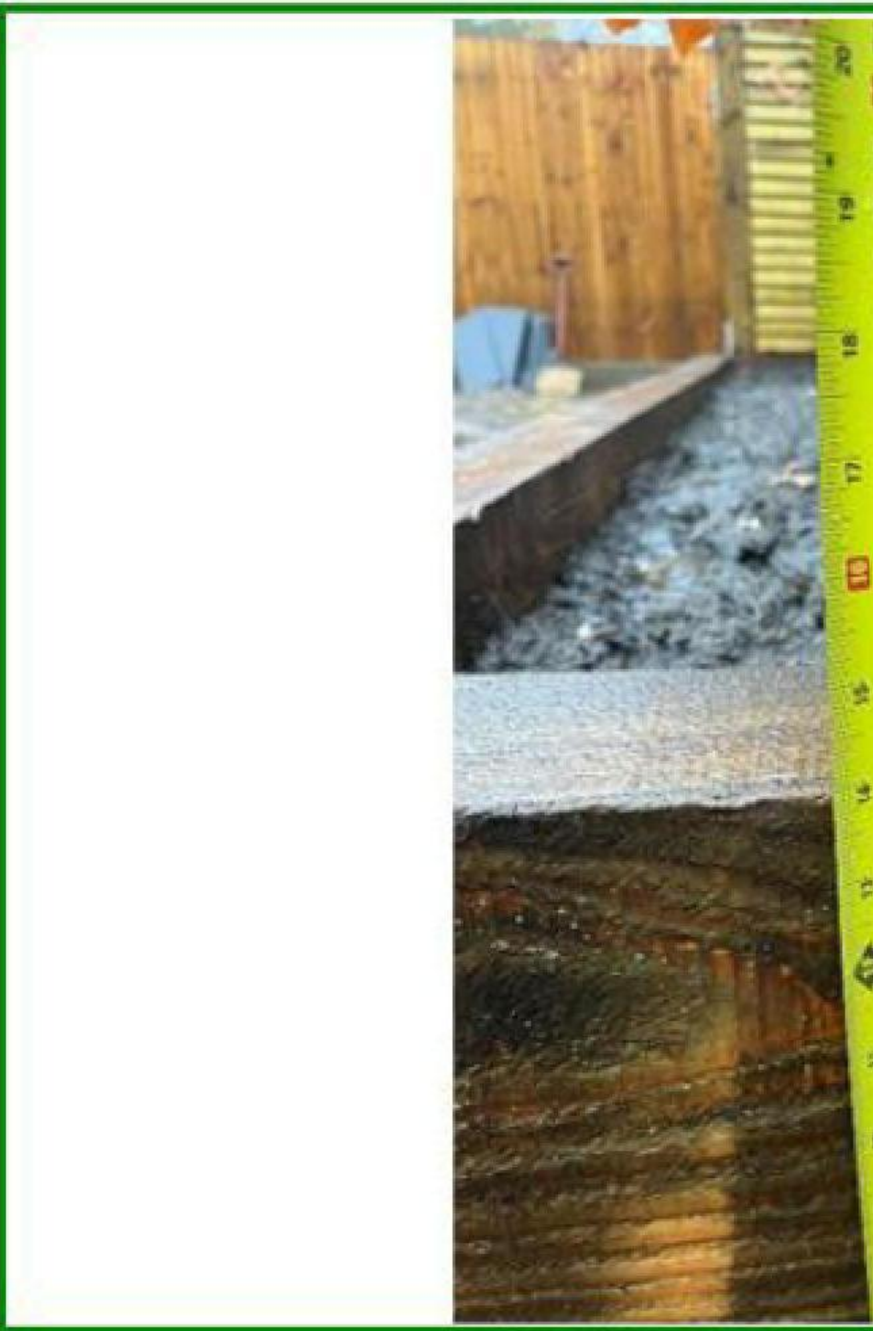
Photo No.4: Depth of raised beds confirmed to be circa 150mm below ground level.
