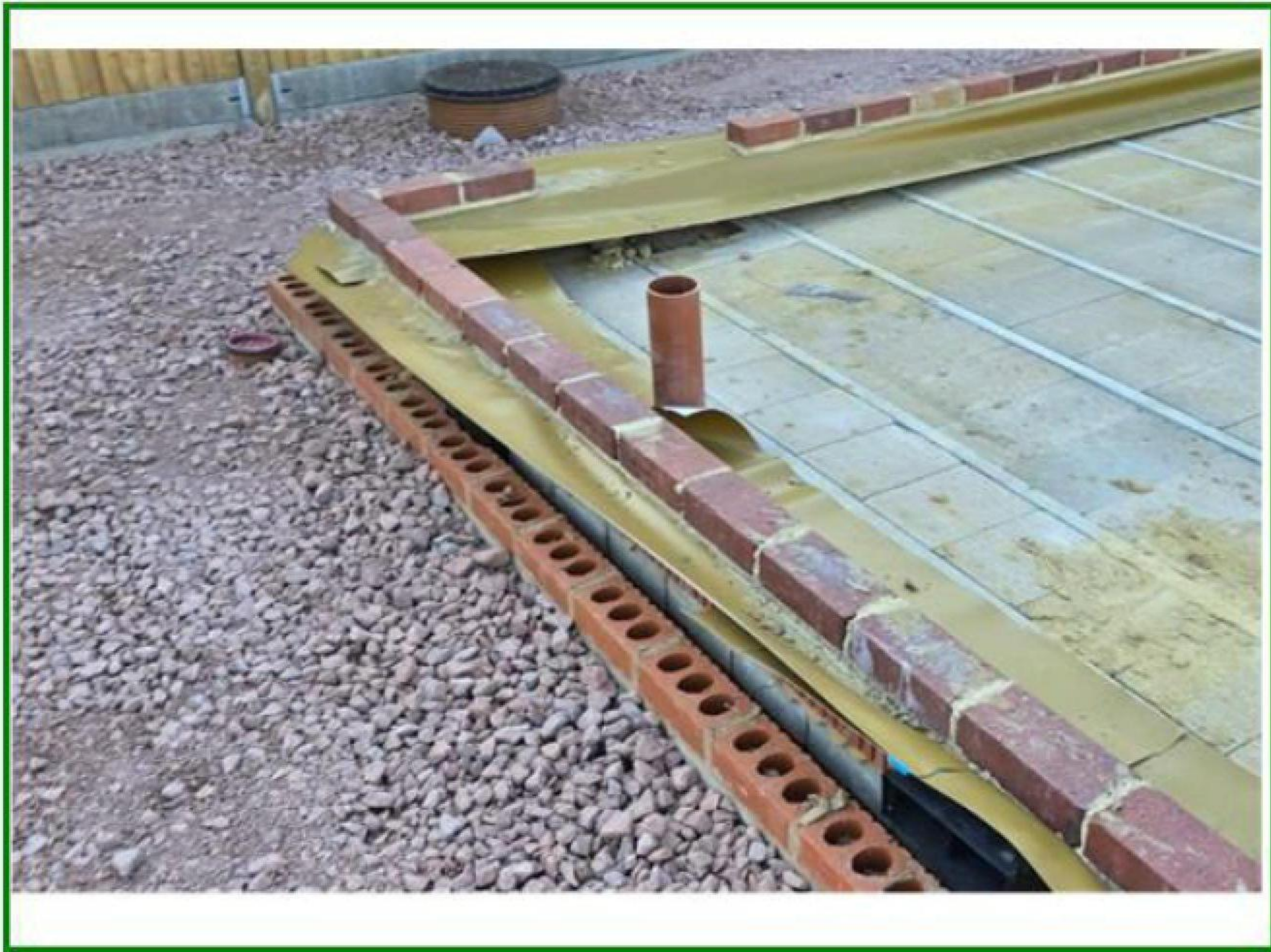
Photo No.7: Beam and block foundation with service penetration and membrane through wall.
