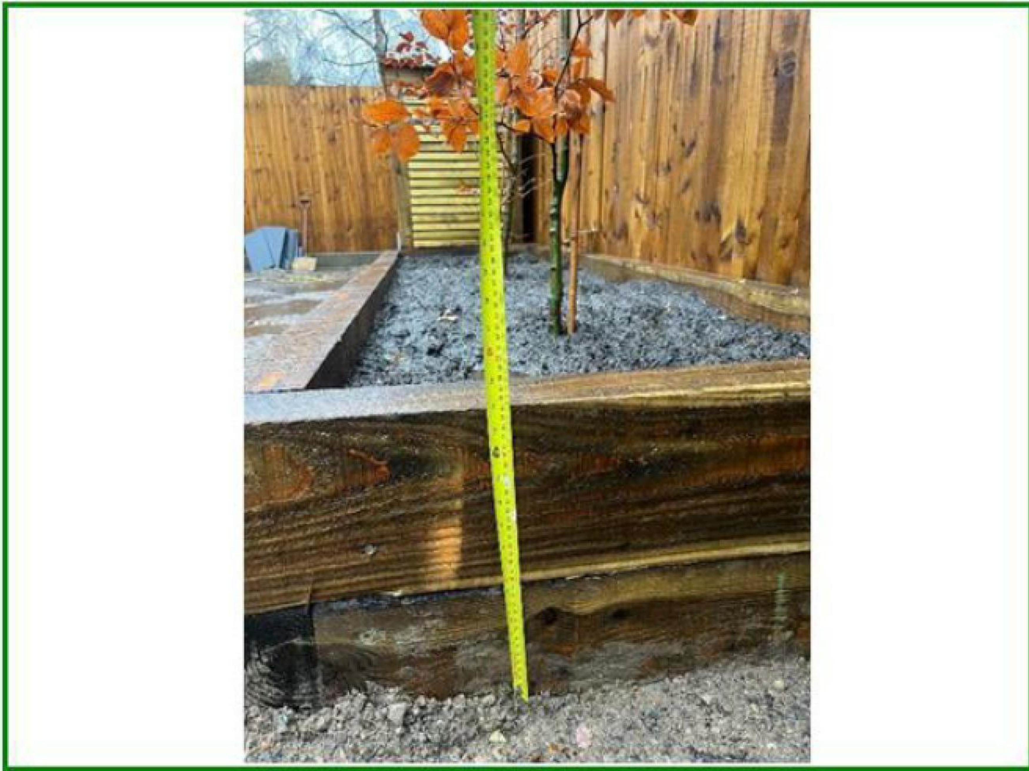
Photo No.3: Height of raised beds confirmed to be circa 360mm above ground level.
