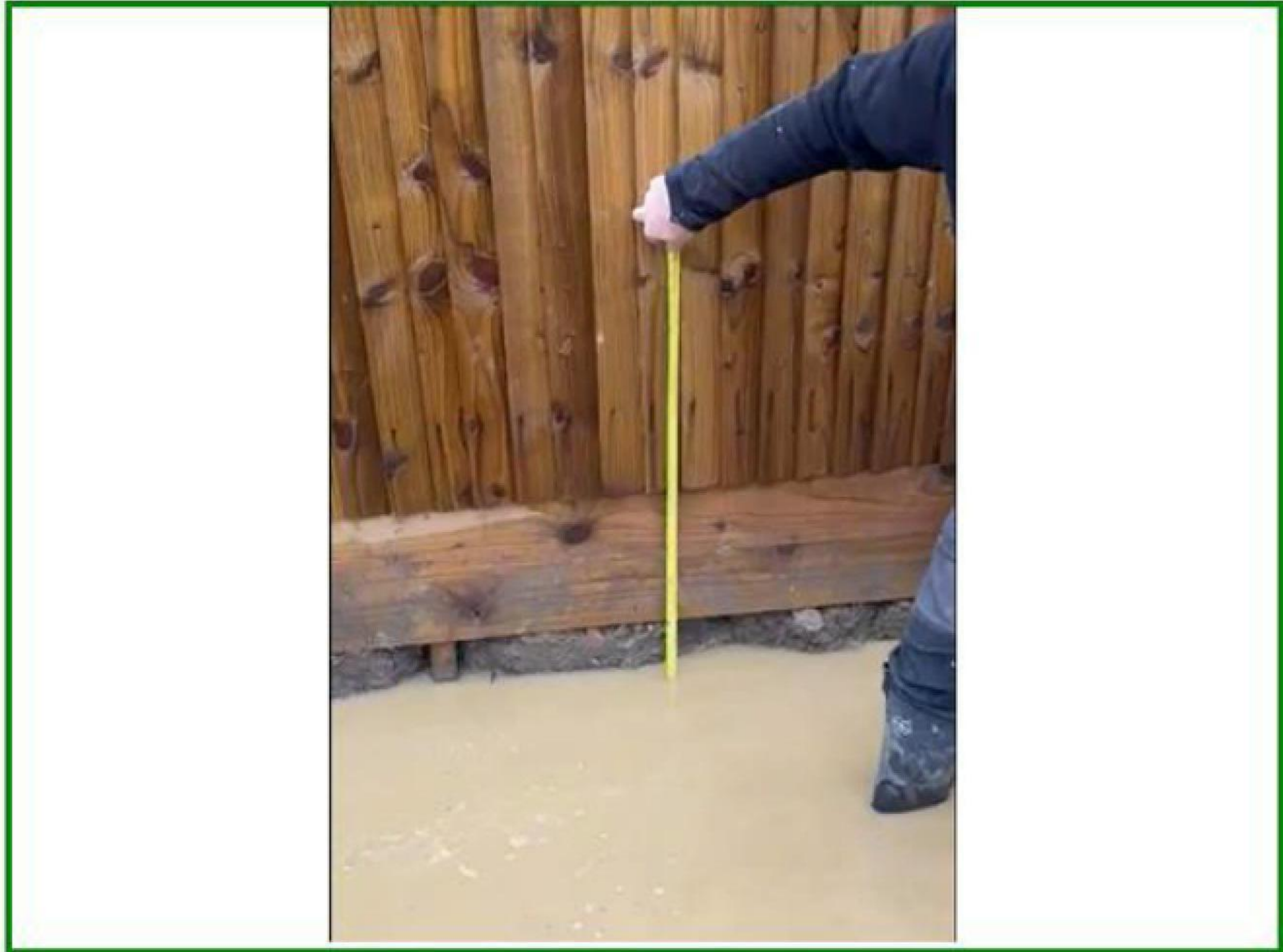
Photo No.1: Excavation in northern site area. Original ground level approximately half way up bottom board.
