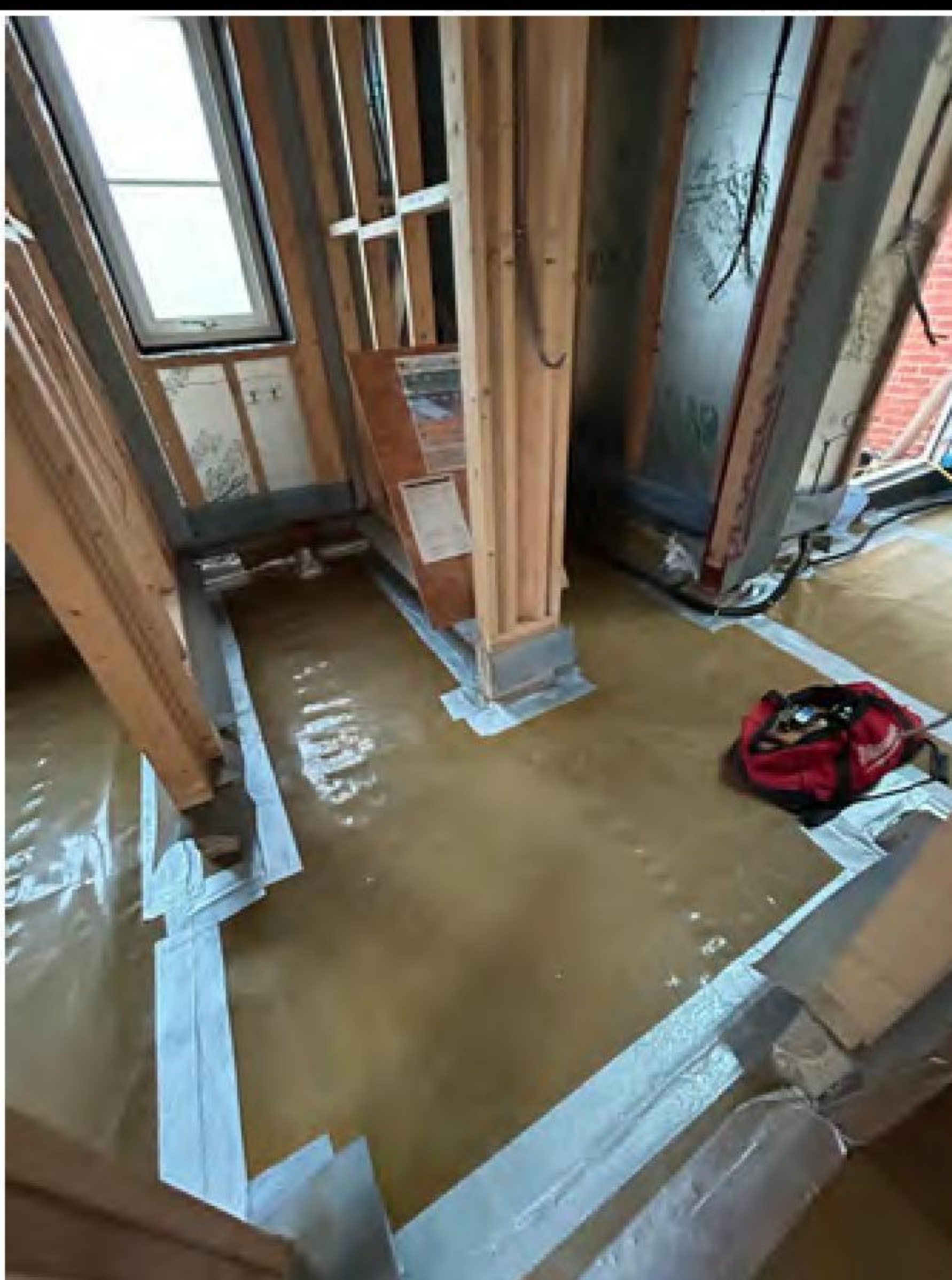
An overview of the infill installation to one of the rooms.
