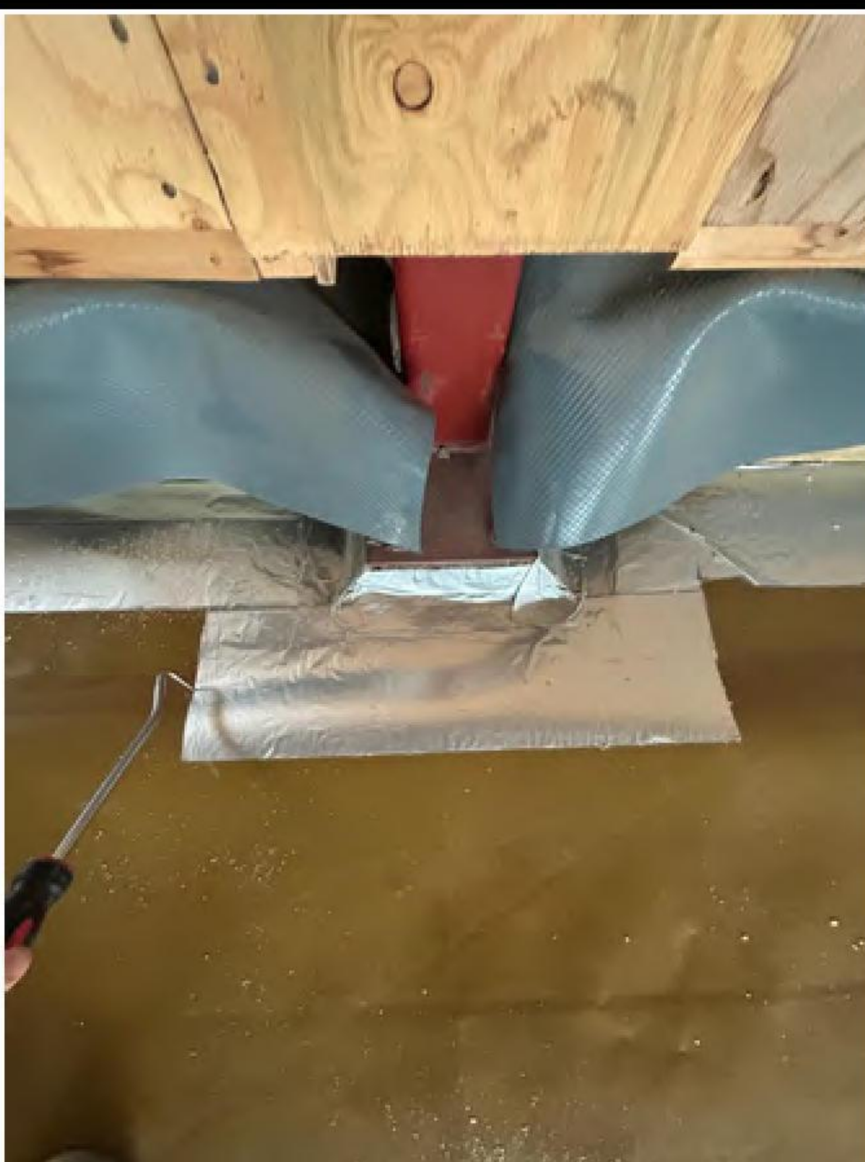
A mechanical point stress test being conducted upon a column, sealed with Visqueen Pro Detailing Strip.
