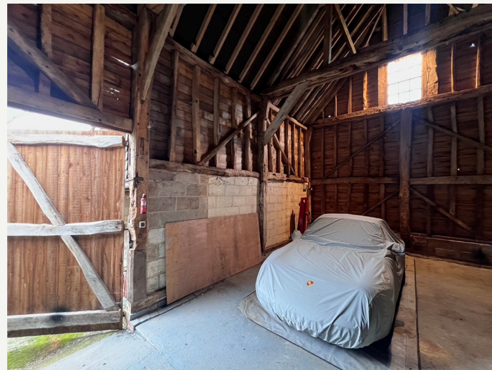
EXISTING BLOCKWORK WALL TO PARTITION BETWEEN CATSLIDE AND MAIN VOLUME
