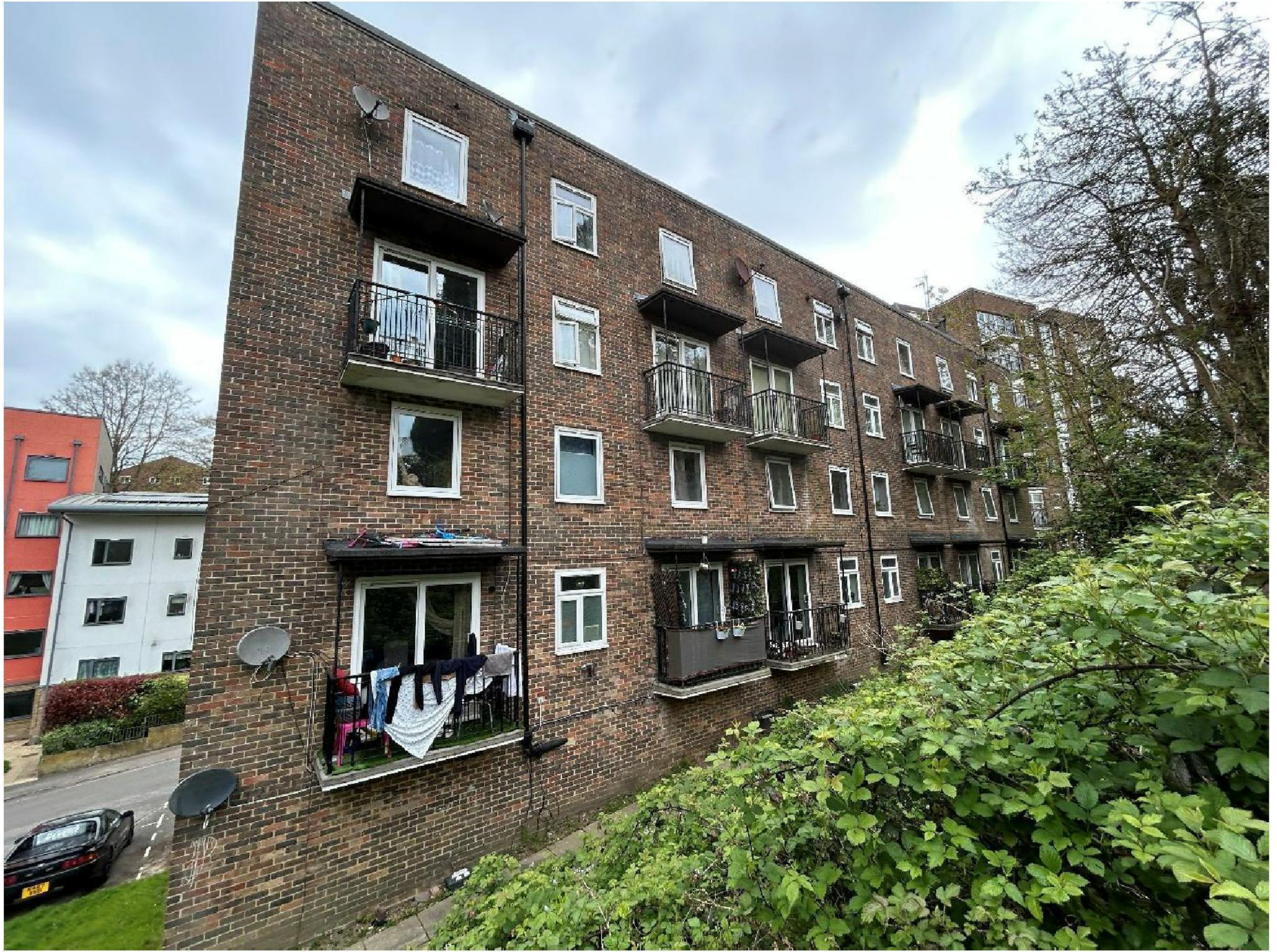
Existing Private balconies.
