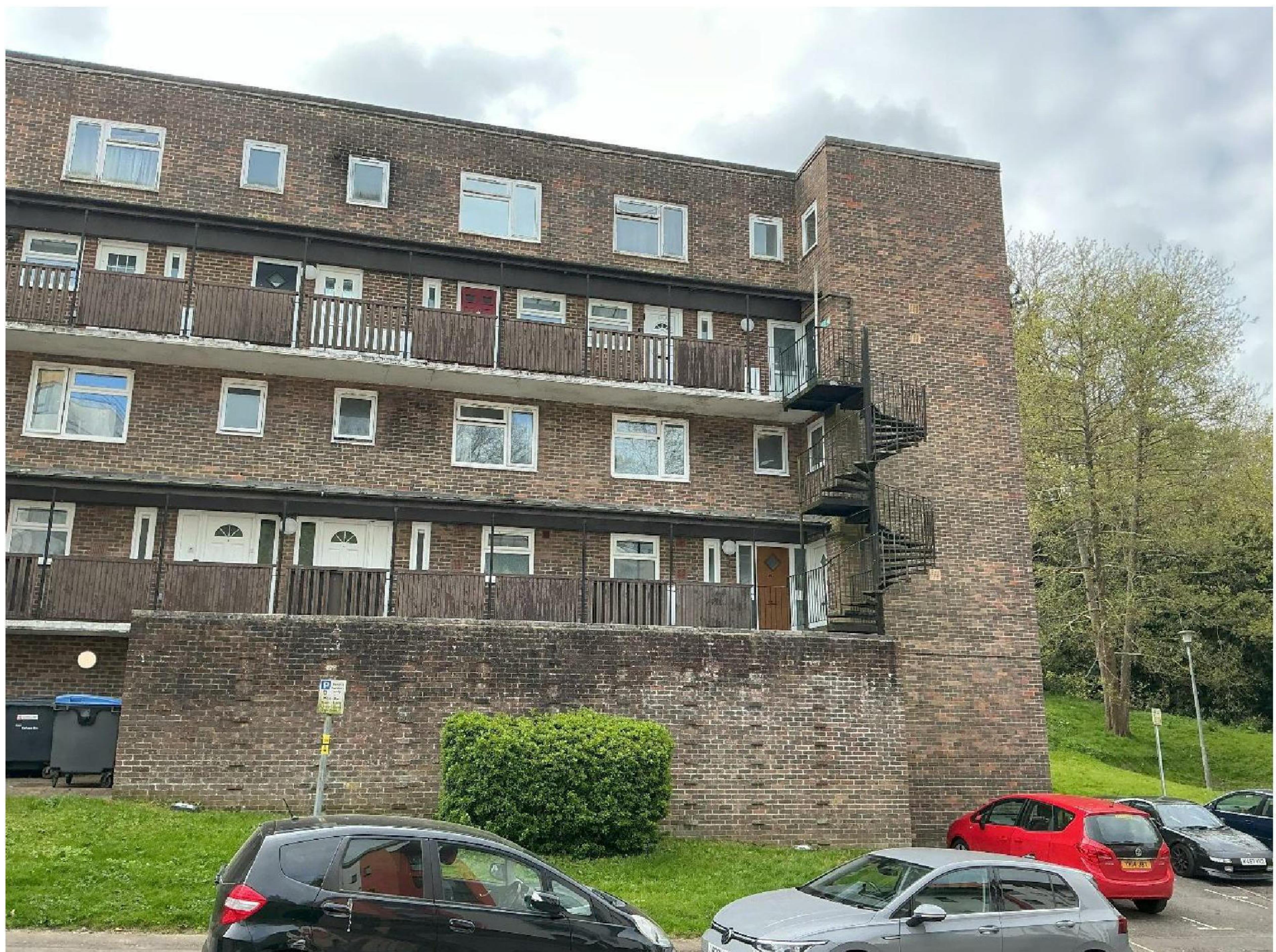
Existing front elevation with front balustrades.
