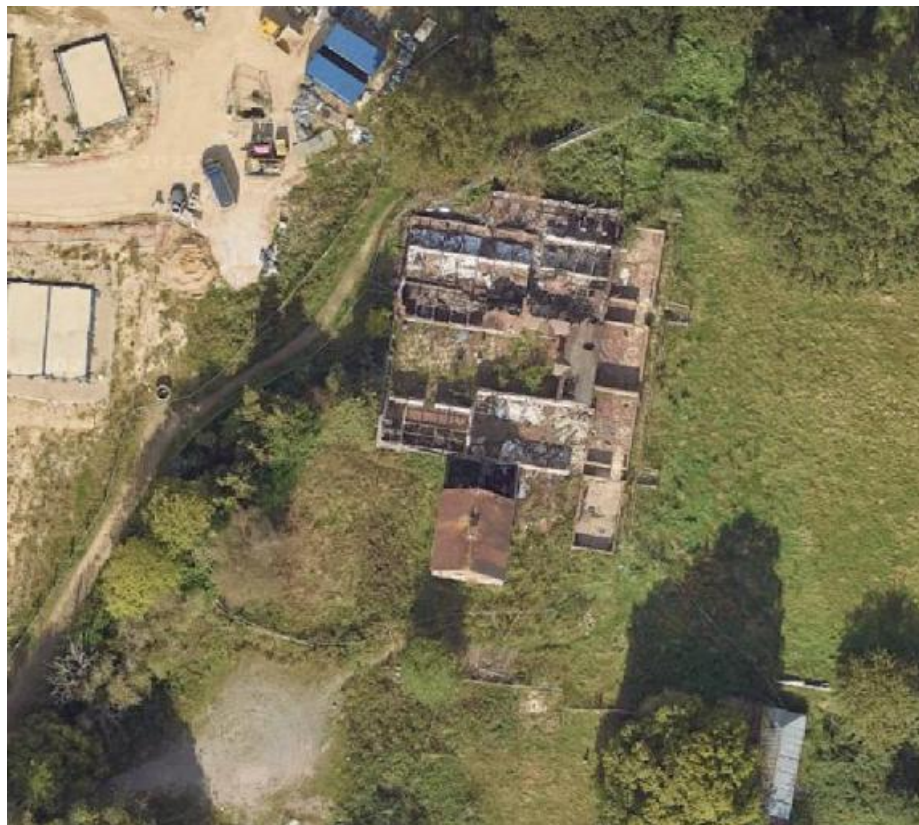
Figure 1. Google aerial image of the buildings that have been significantly damaged by fire ( NB in the below image, B1 that supported the maternity roost is still present although now, the roof has been lost to fire damage (happened in 2024), B4 and B5 are no longer present as well )
