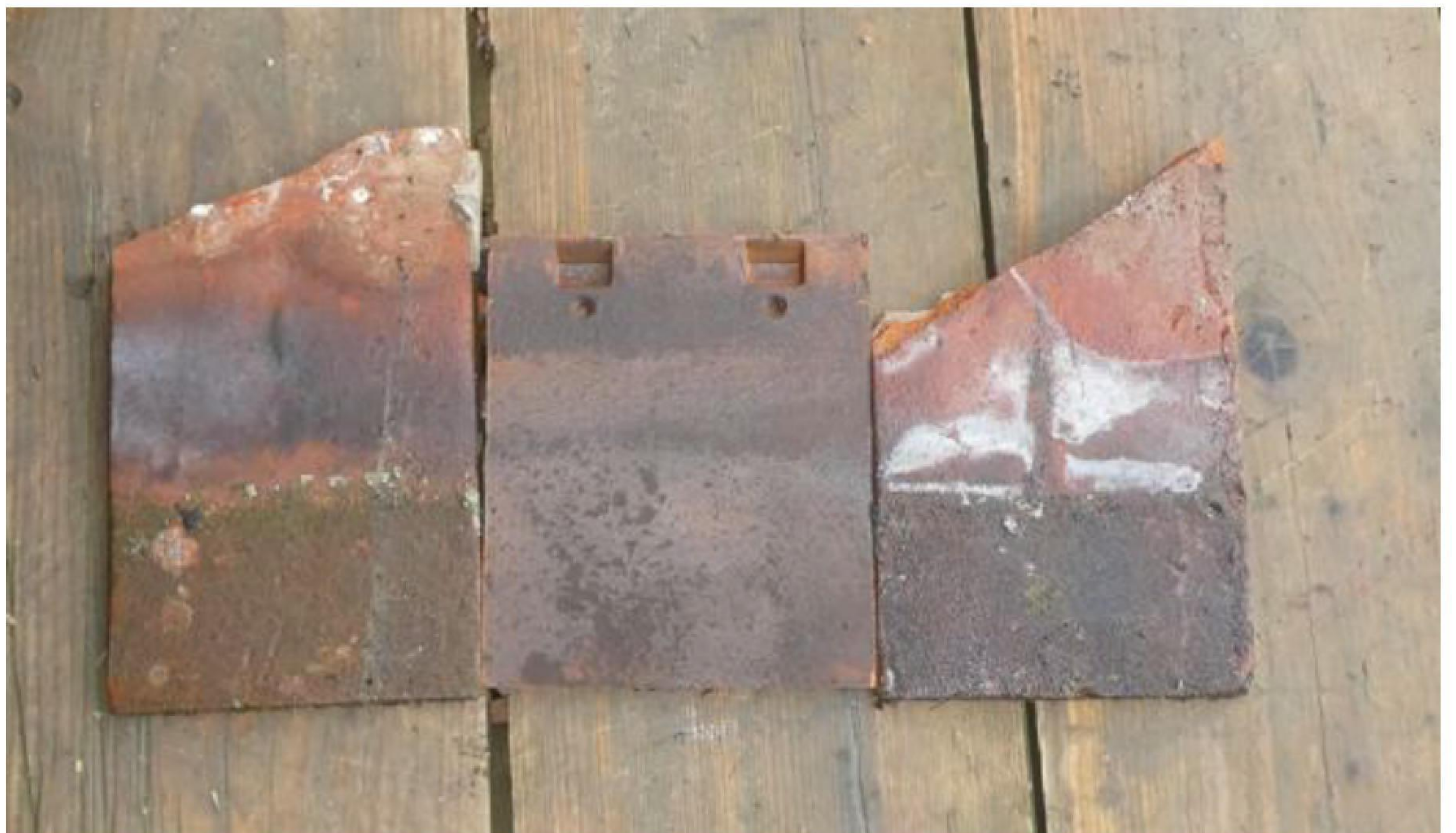
Edilans Phalempin Weathered Plain tile laid between two original removed tiles
