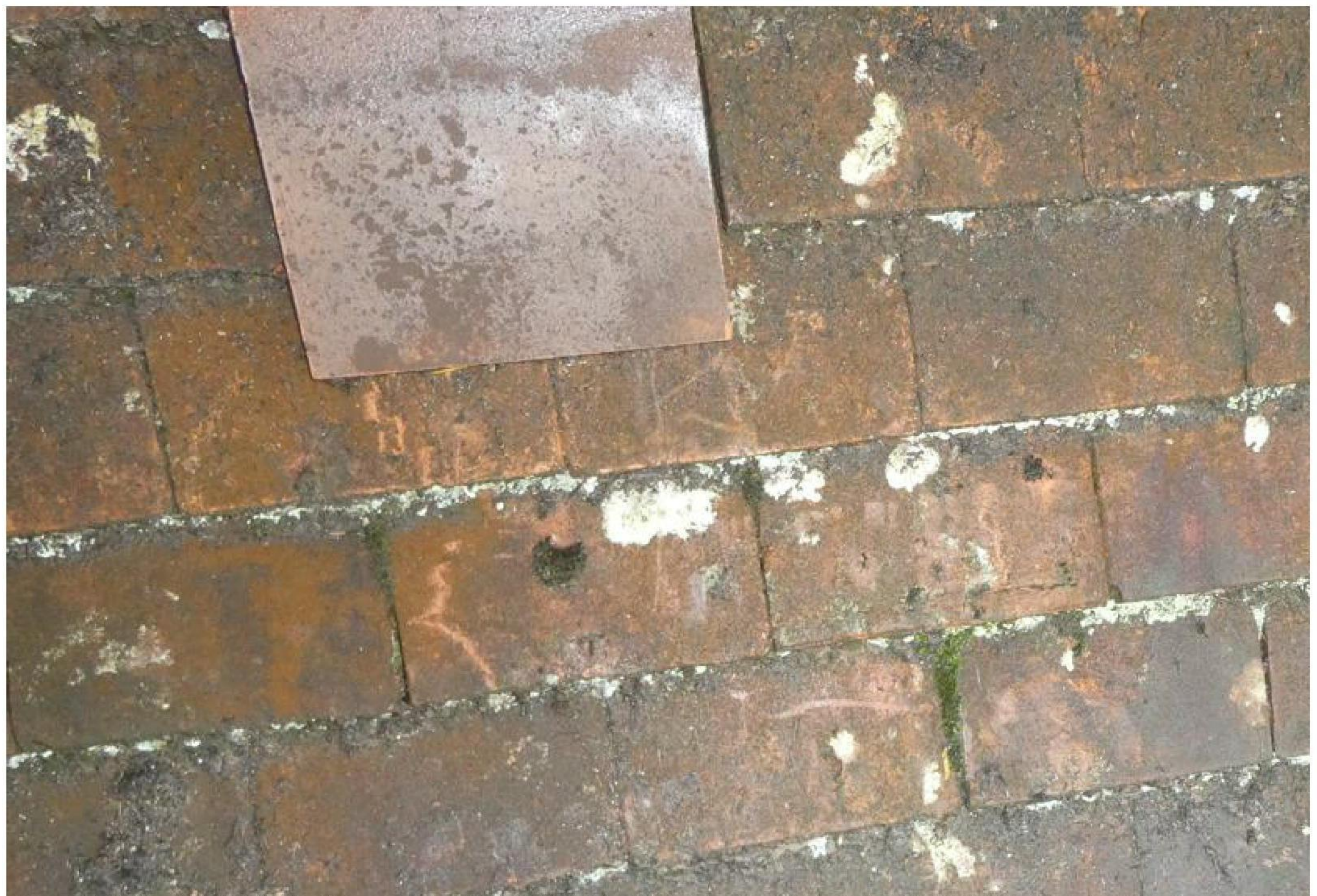
Edilans Phalempin Weathered Plain tile laid on existing The original tiles are a closer match when clean
