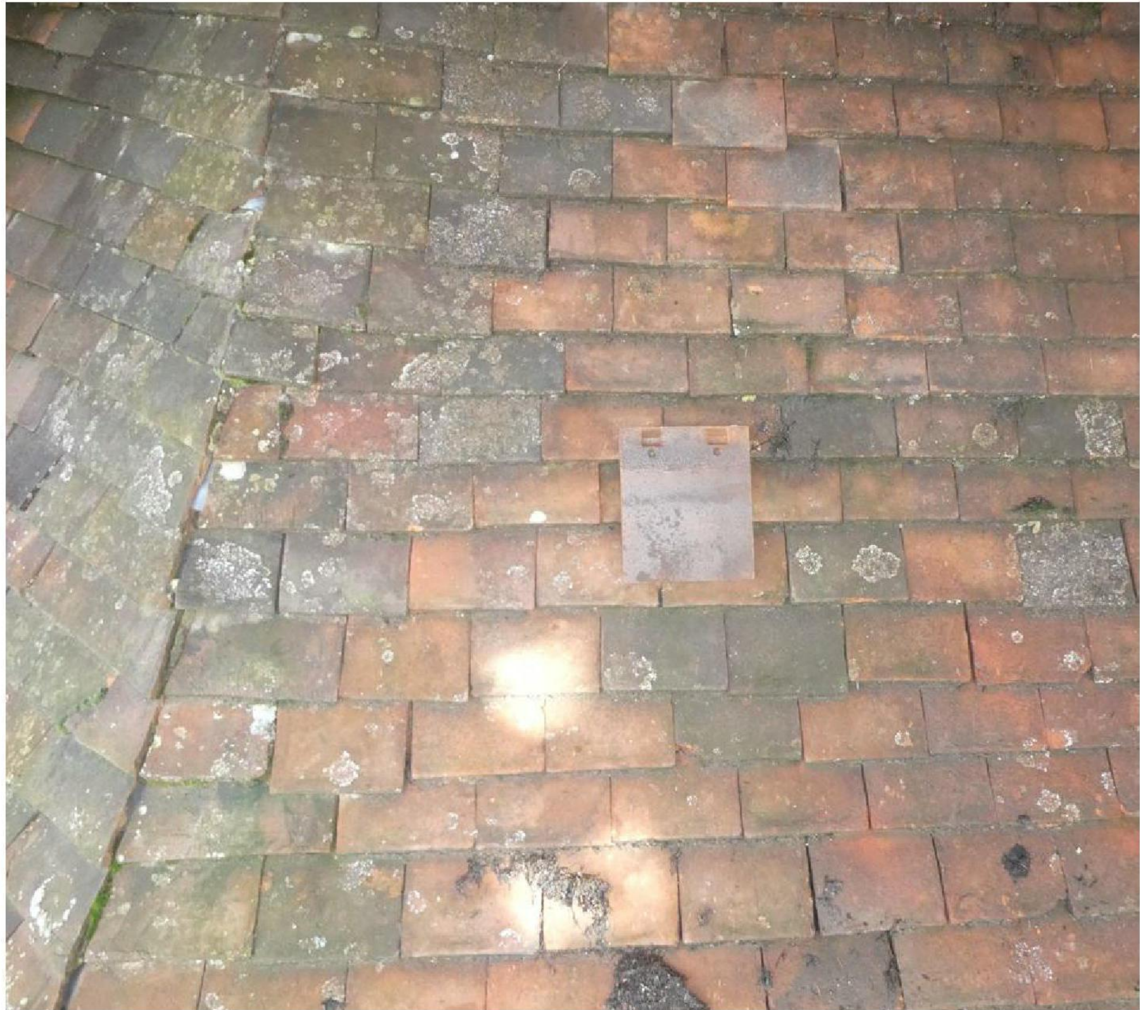
Edilans Phalempin Weathered Plain eves tile showing colour match Mitred tile to external corner
