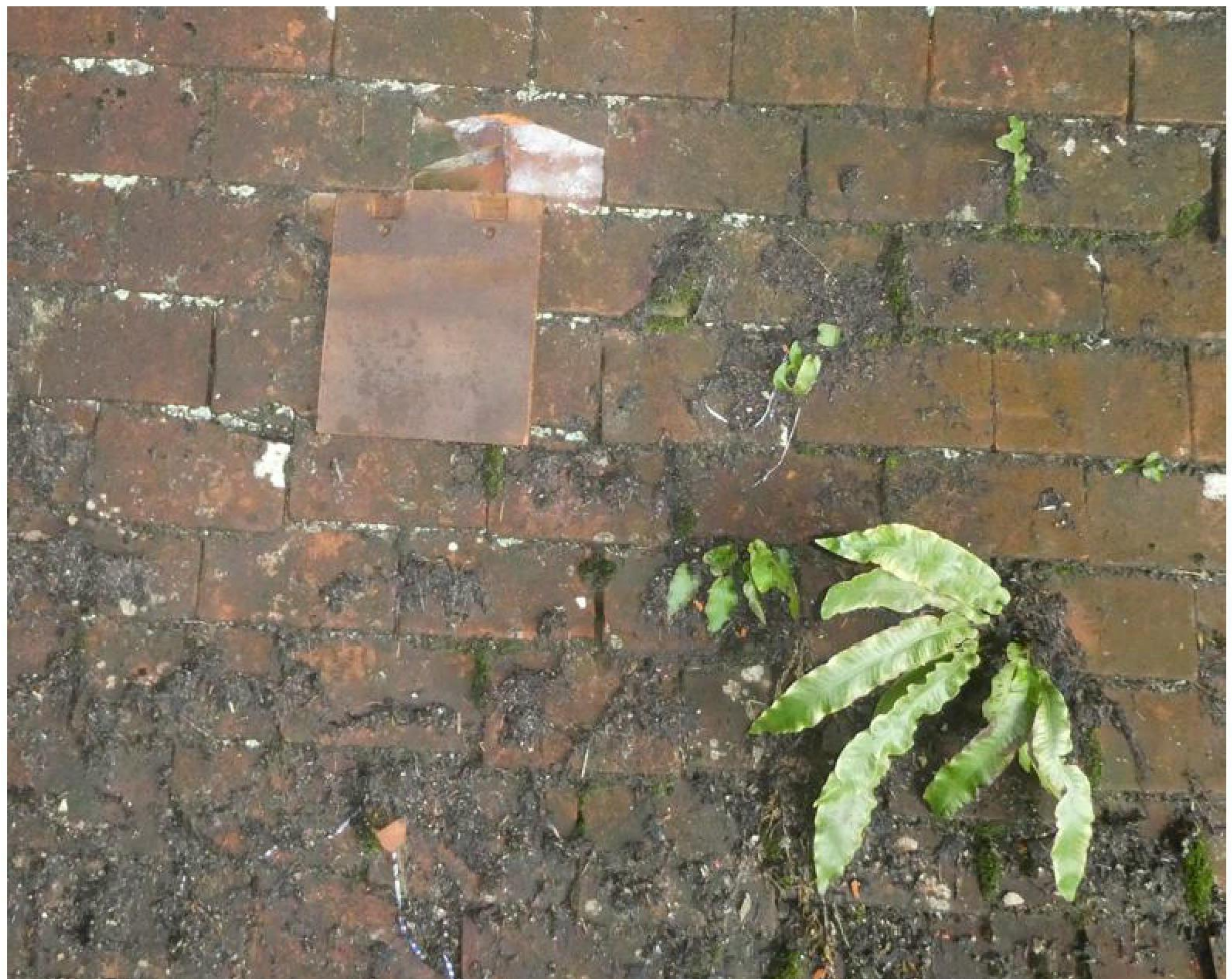
Edilans Phalempin Weathered Plain tile laid on low pitch section of roof
