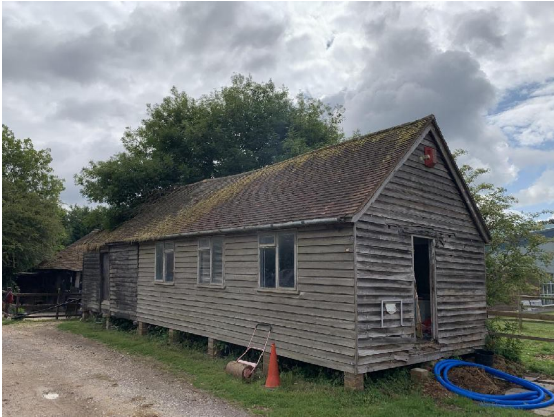
Photograph 3: Overview of the building to be demolished.
