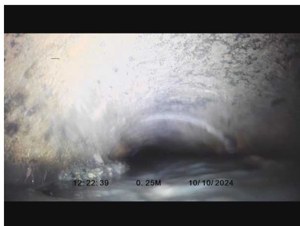
2, 00:00:07, 0.00 m Water level, 10% of the vertical dimension
