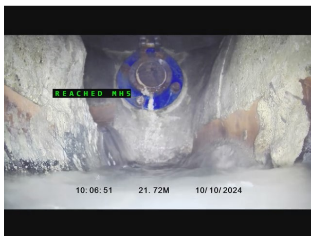
4, 00:01:13, 21.72 m Finish node, manhole, reference: MH5
