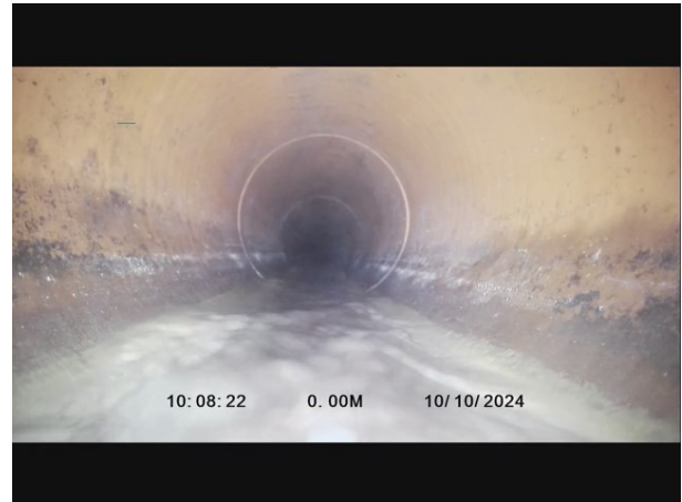
2, 00:00:04, 0.00 m Water level, 5% of the vertical dimension
