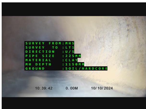
1, 00:00:00, 0.00 m Start node, manhole, reference: MH5
