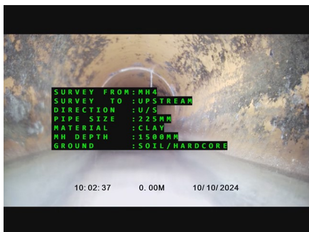
1, 00:00:00, 0.00 m Start node, manhole, reference: MH4
