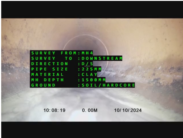
1, 00:00:00, 0.00 m Start node, manhole, reference: MH4
