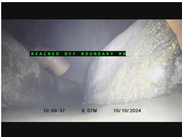
5, 00:00:50, 8.07 m Finish node, manhole, reference: Off Boundary Manhole
