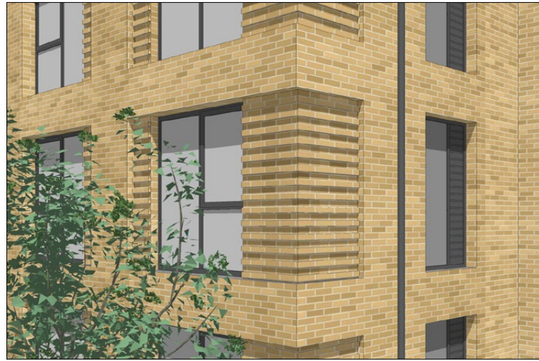
TEXTURED BRICKWORK PANELS
