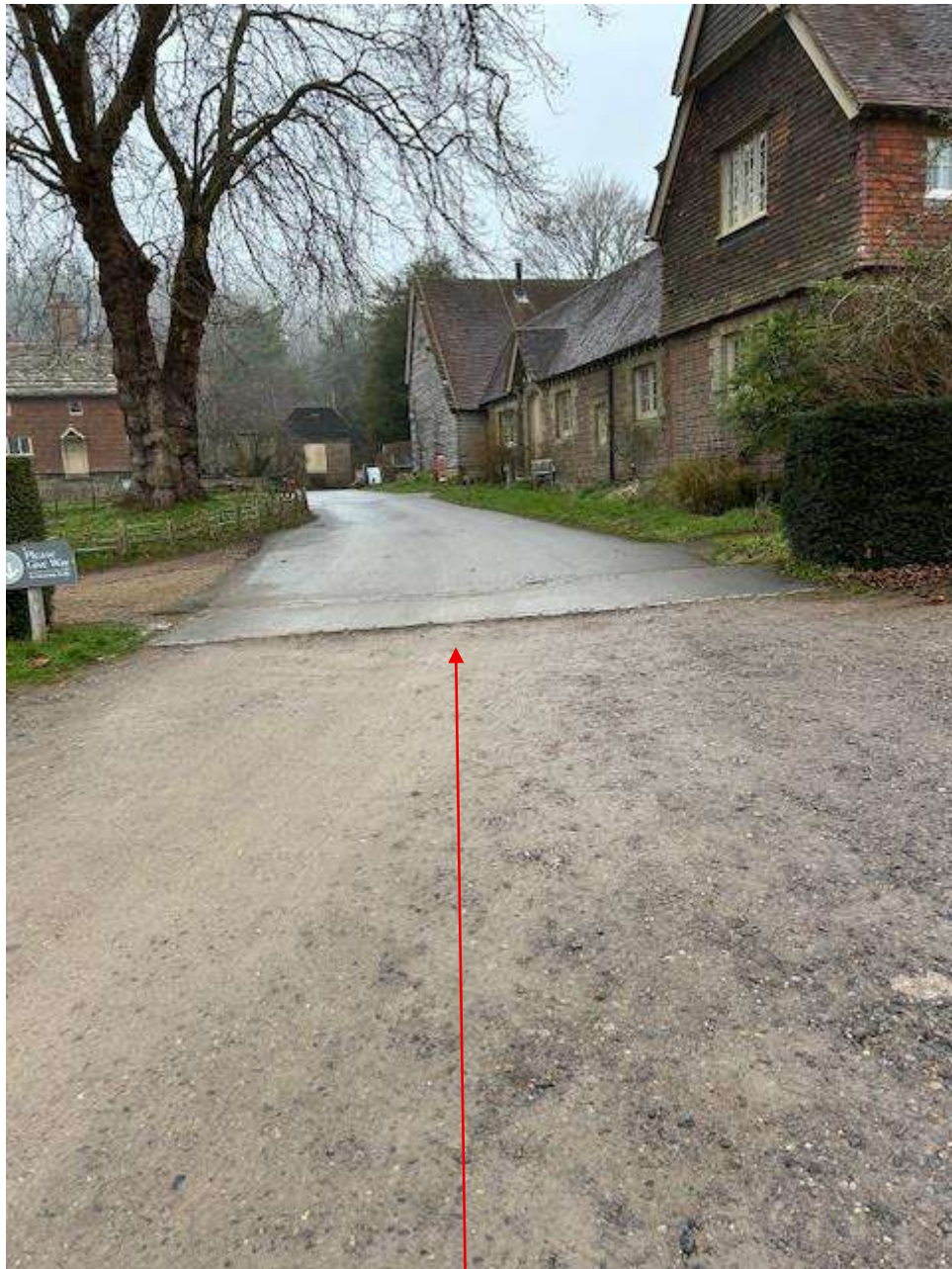
Photograph 2 – Section of main access drive where surfacing changes from tarmacadam to crushed stone adjacent to the Barn Cafe.
