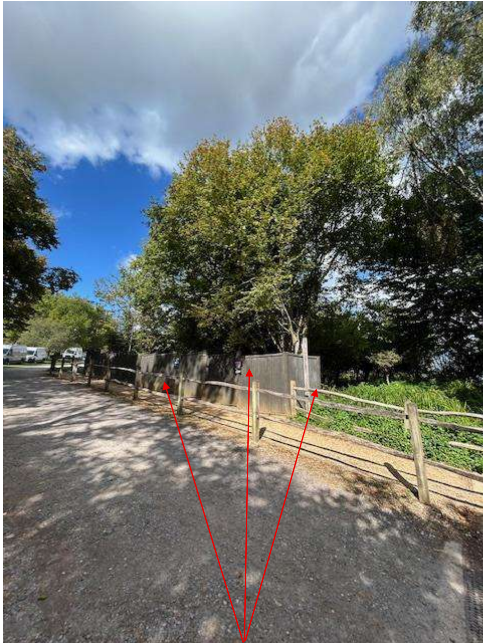
Photograph 7 – Section of wooden post and rail fencing and close board fencing on northern side of path and wooden post and rail fencing on southern side of path.
