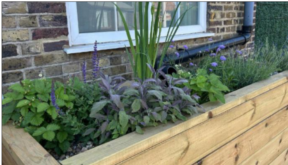
Figure 4.2 SuDS Planter installation (Meristem Design 2026)
