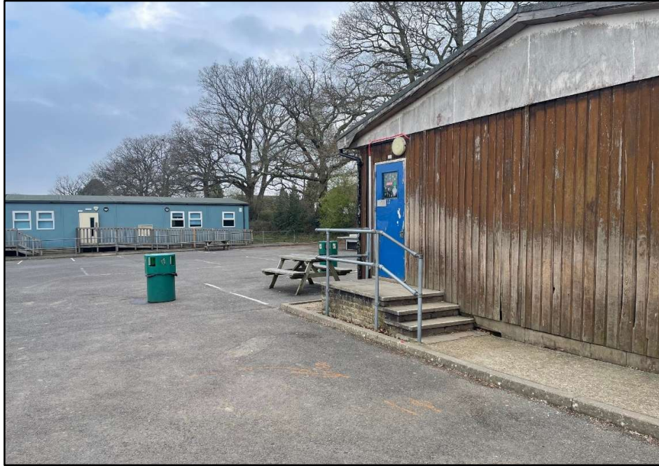
Figure 2 Looking North within the application site. The music classroom building is to the right of the picture.
