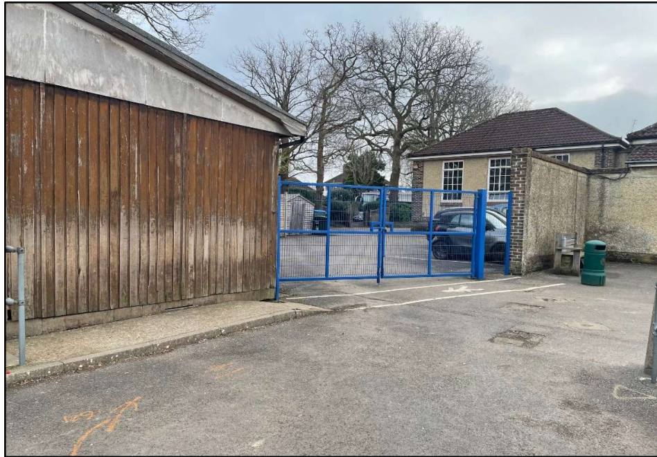
Figure 4 Looking south east within the application site. The music classroom building is to the left of the picture.
