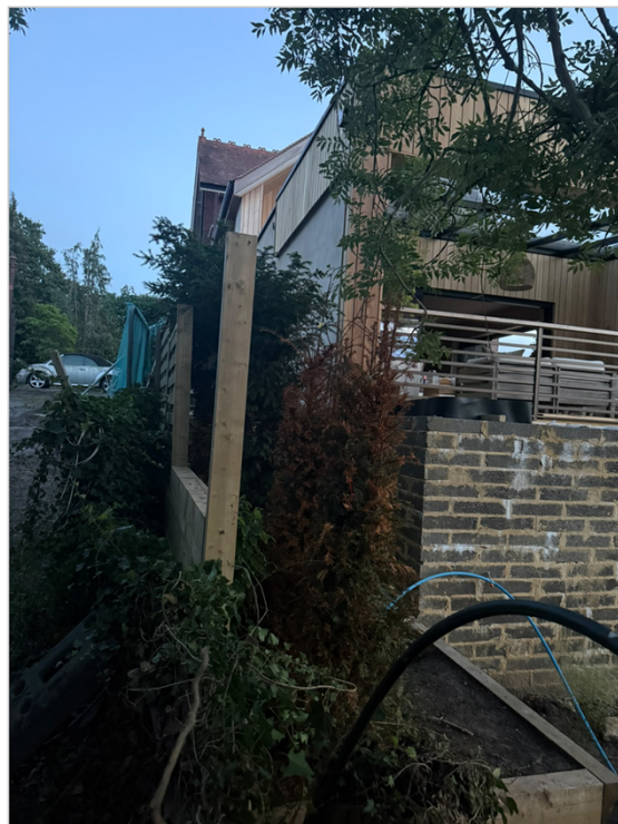
Photo 2 — The same boundary viewed along its length, showing how close No. 44's living accommodation sits to the line the track would follow. The applicant's hedge, fence, track and the ash's root protection zone must all share this strip.
