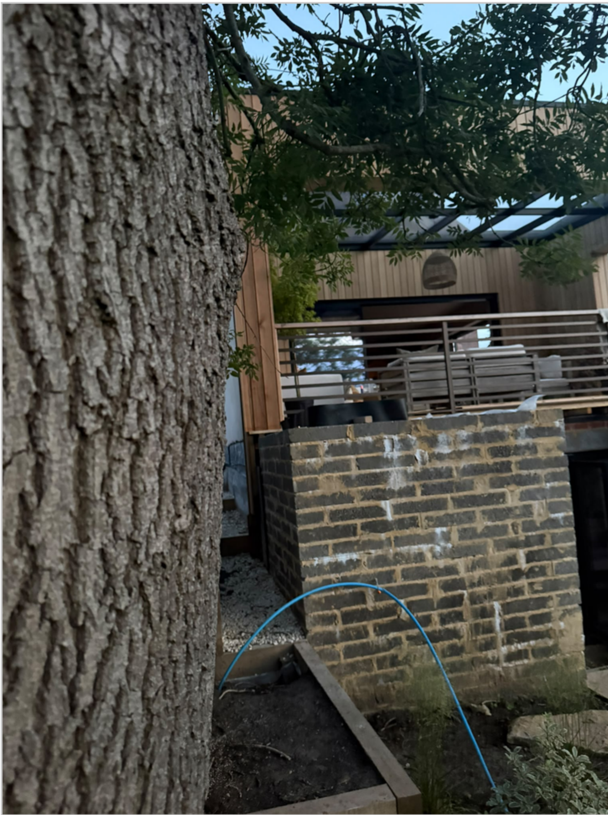
Photo 1 — The boundary ash — the tree for which the Tree Officer records no root protection calculation — with No. 44's outdoor dining area, kitchen and bedroom immediately behind. The ash stands on the shared boundary: the proposed 32-metre access track would pass on its far side, a few feet from these rooms. (The blockwork is No. 44's own wall, awaiting cladding.)
