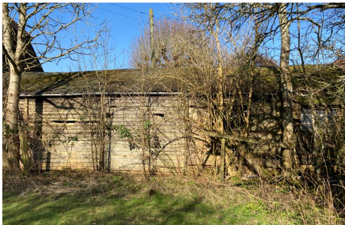
Modern building replacing the historic range to the east of the barn.
