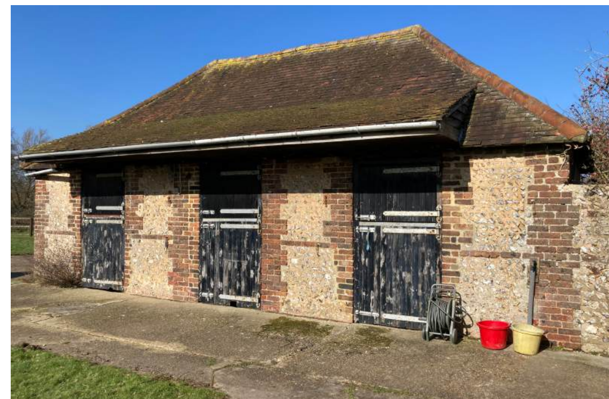
South elevation of the stables. Note the altered doorways and eave to form canopy.
