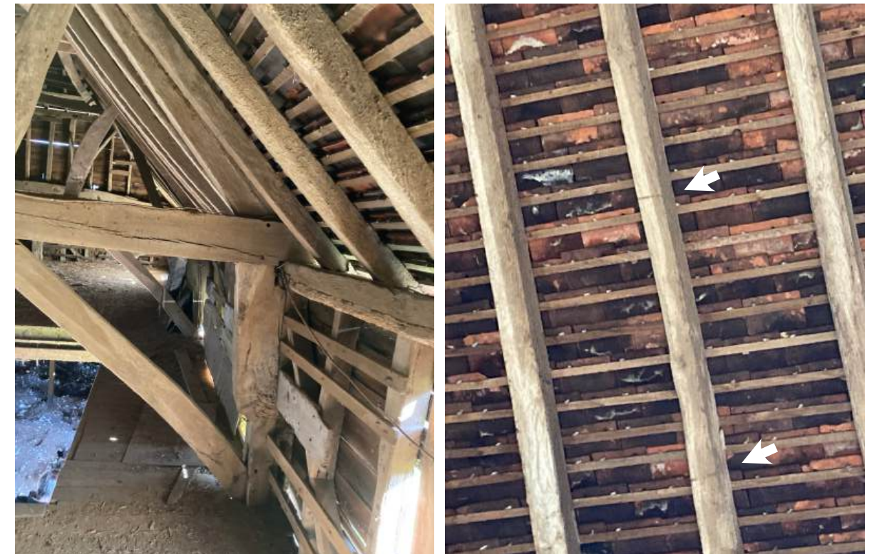
Late 17 th century jowled post and curved brace (left) and tar marked rafters indicating a former thatched roof (right)
