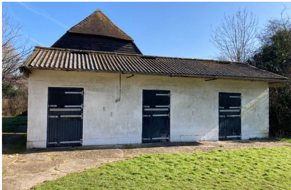
Modern outbuildings to be replaced.
