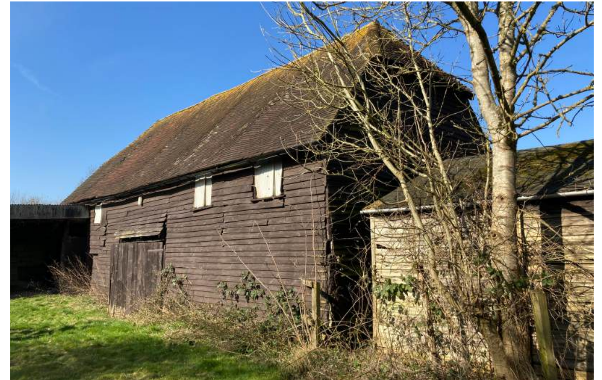
South elevation of the barn.
