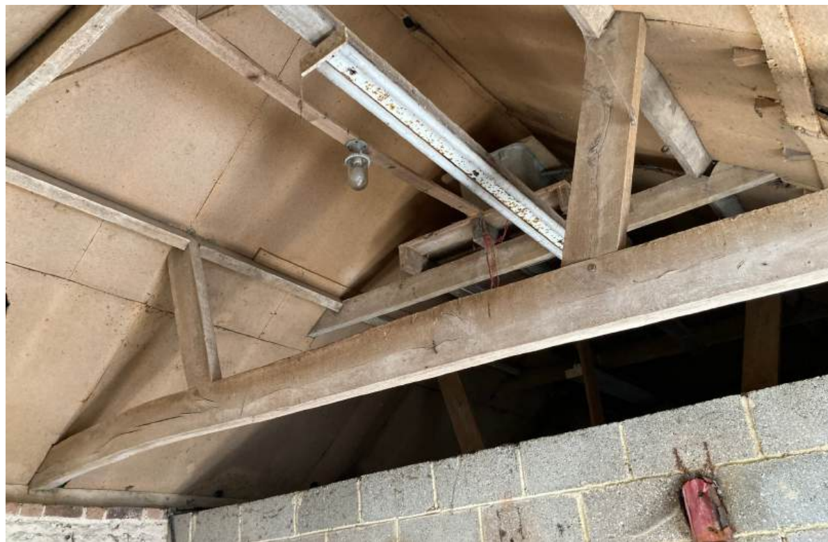
Roof structure of the stables.
