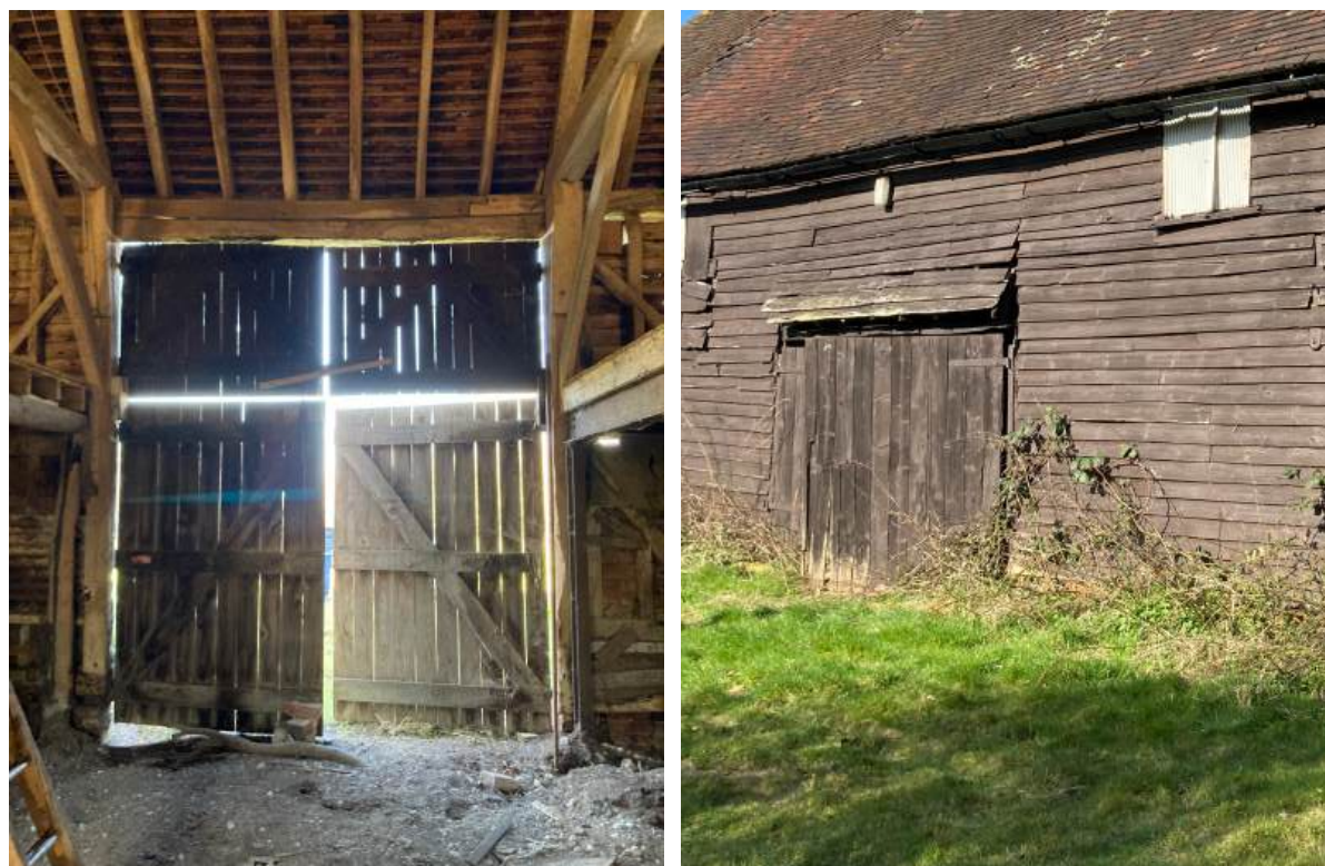
Original main threshing opening (left) and secondary threshing opening (right).
