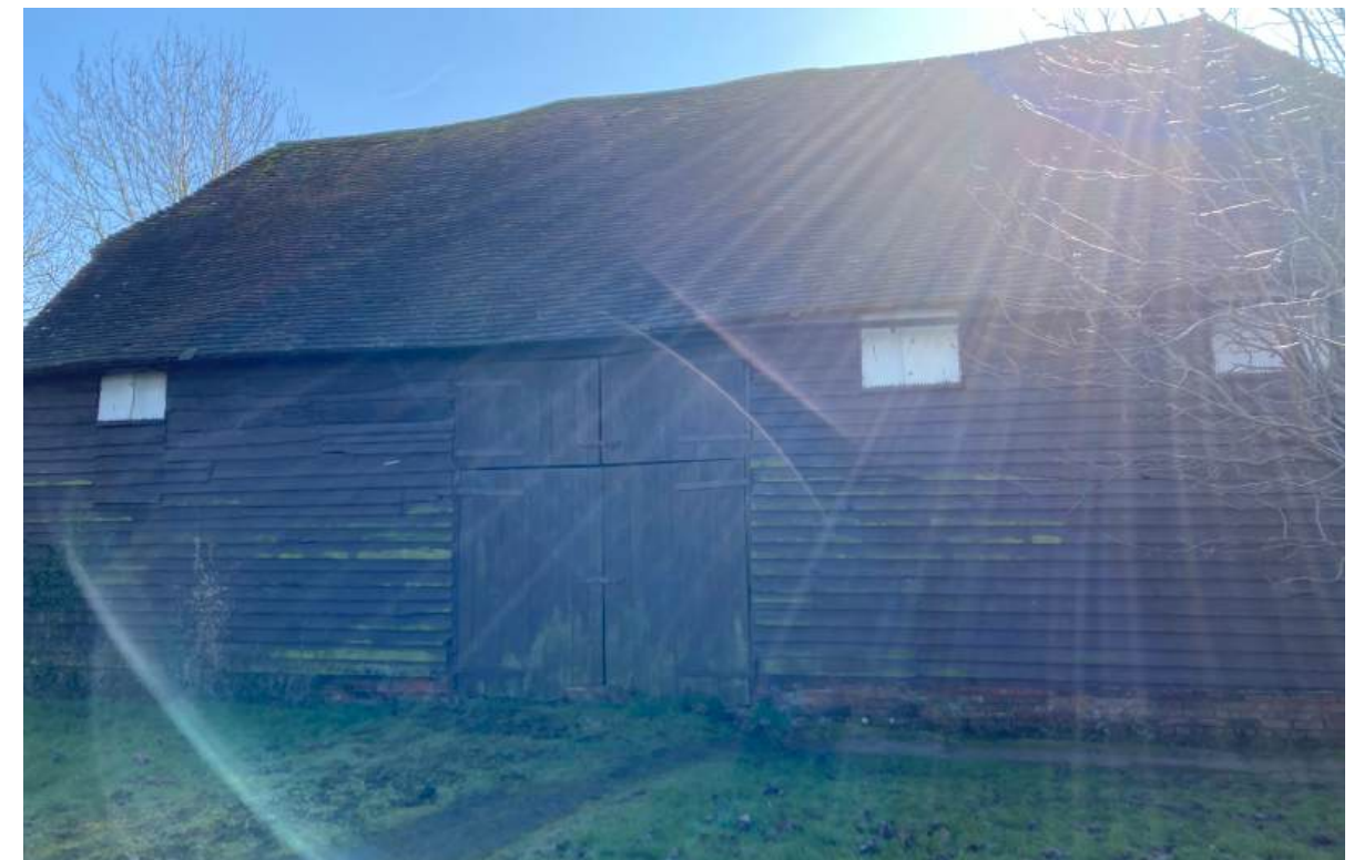
East elevation of the barn.
