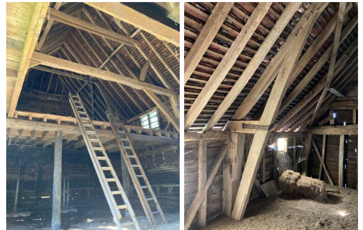
Later inserted mezzanine (left) and sling brace (right).
