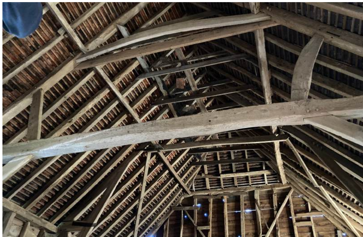
Original late 17 th century truss displaying curve raking struts and side purlins.
