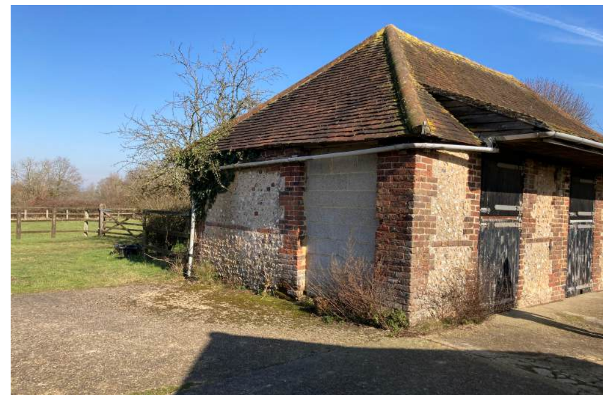
North and west elevations of the barn.
