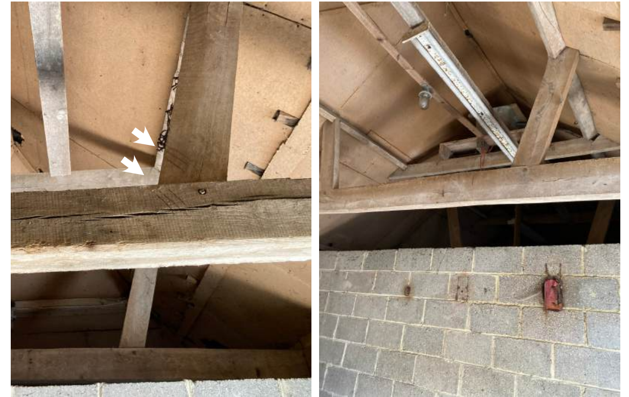
Carpenters' marks (left) and modern blockwork partition (right).
