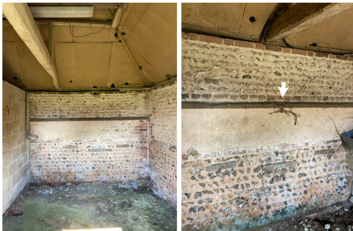
Interior of standing stall (left) and evidence of former manger (right).
