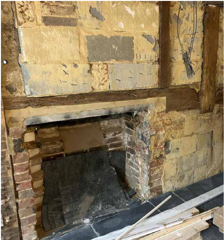
Ground floor living chimney breast prior to re-facing
