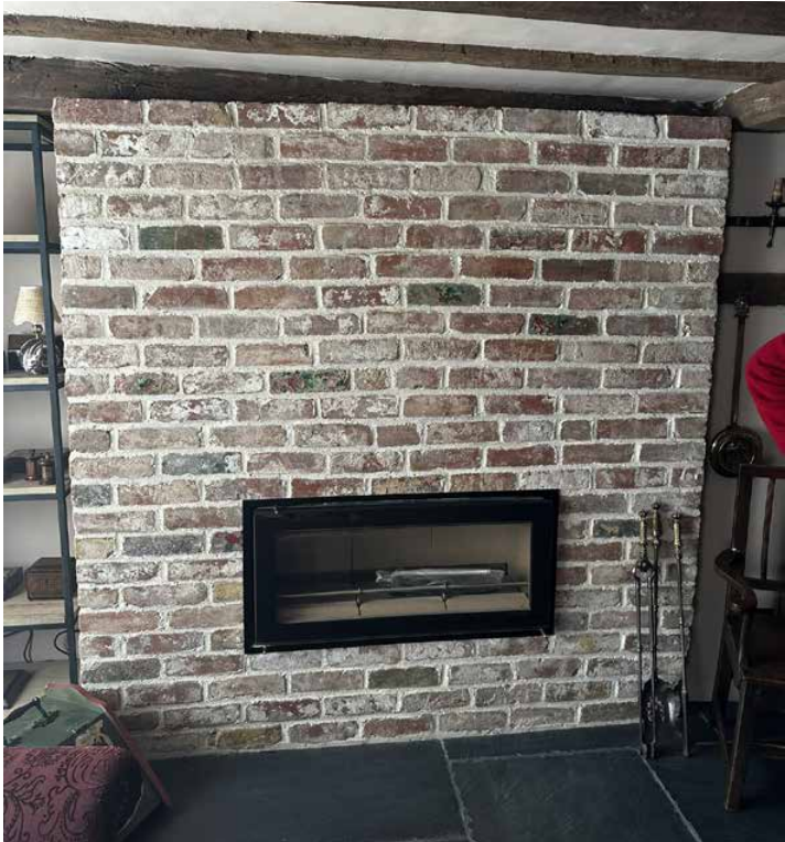
Ground floor living room re-faced chimney breast
