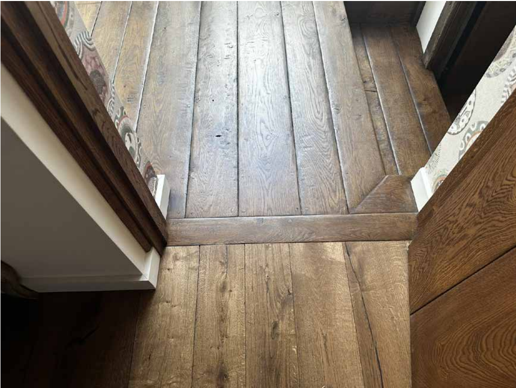
As-built oak flooring
