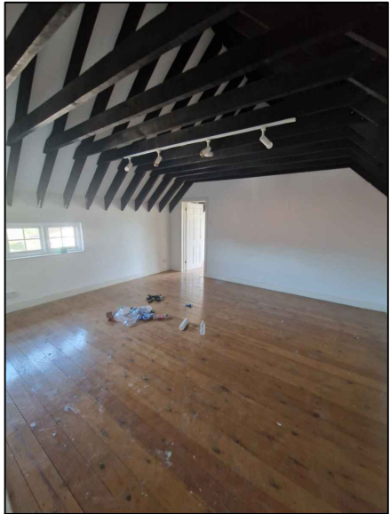
Interior photo of existing ceiling in former annexe (area 1a)
