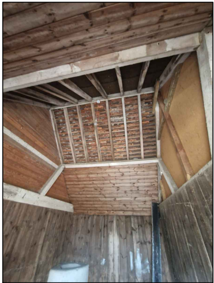
Interior photo of existing ceiling in former stable (area 1b)
