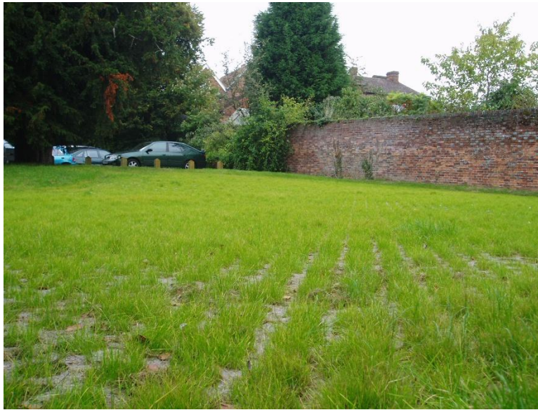
Figure 2: Example of grasscrete system.
