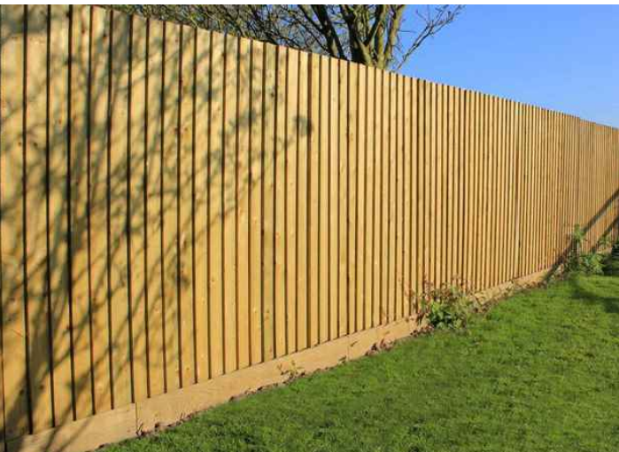
2.0m Close-boarded timber fencing with gravel board
