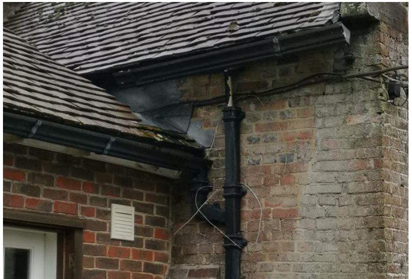
Rainwater Goods House – Black Cast iron, profiles to match existing Extension – Metal
