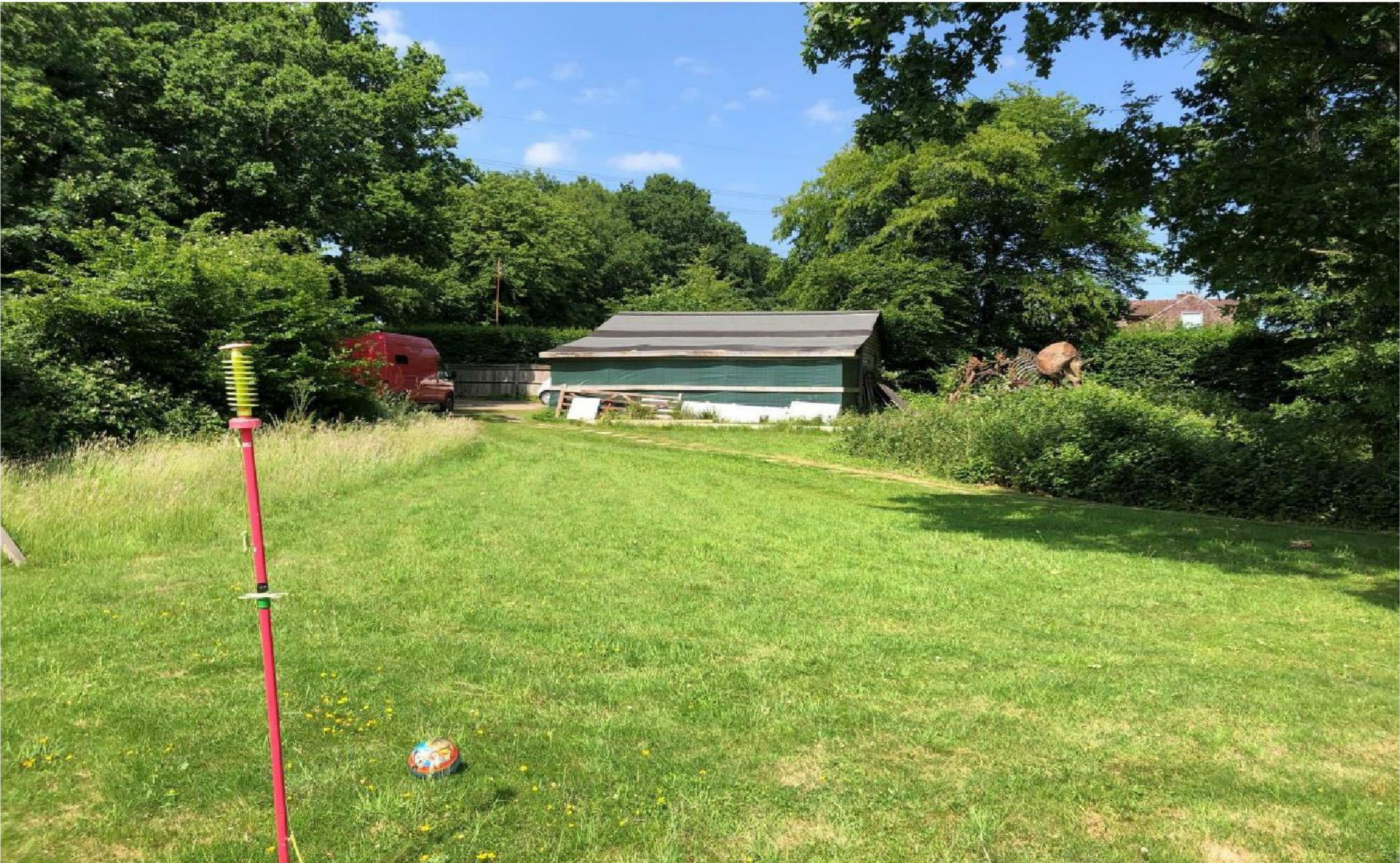
Photo No. 2: - Displaying the modified grassland and garage building (B2) to be demolished within the proposed construction zone.
