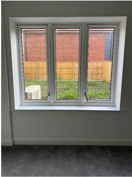
Photo 5 - Example of compliant Living Room window depth and handle height
