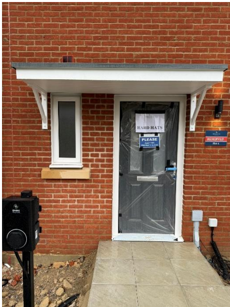
Photo 2 - Example of compliant entrance with level landing, level threshold, canopy and light
