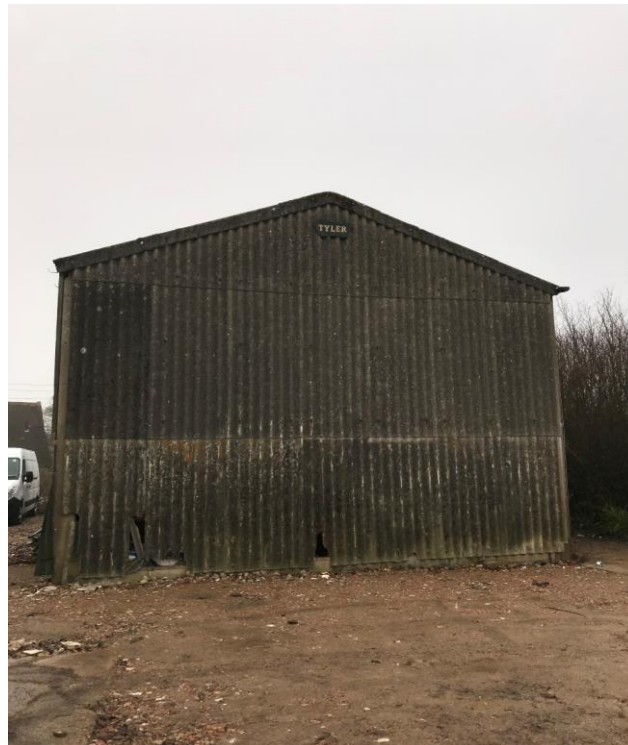
Photograph 18: View of one of the buildings located in the south east of the Site, which is likely clad with corrugated asbestos panels.
