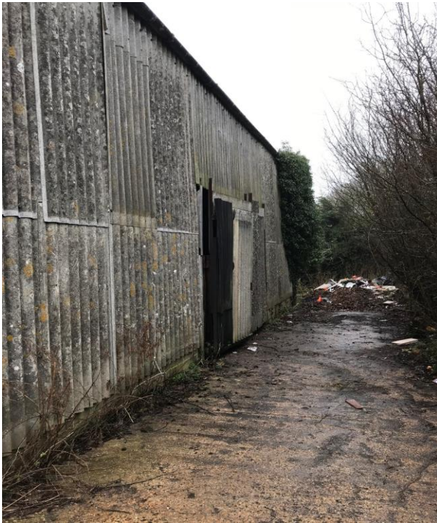
Photograph 19: View down the side of the building located in the south east of the Site, which is likely clad with asbestos.
