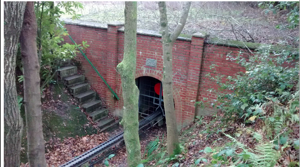
Photo 8 – Miniature railway tunnel/cutting to the SE of the overgrown area
