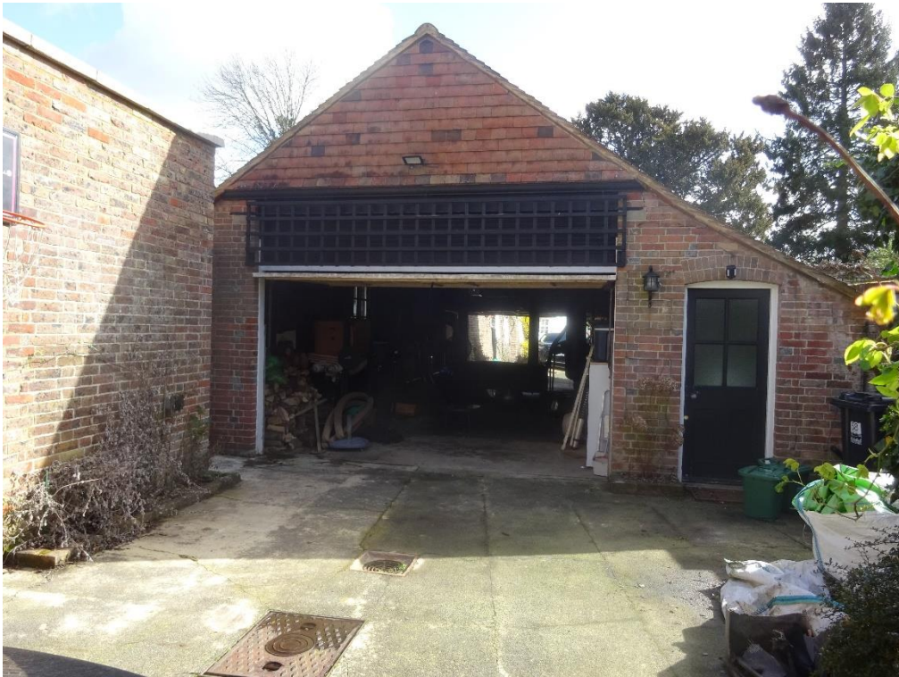
Figure 4 View of garage from driveway
