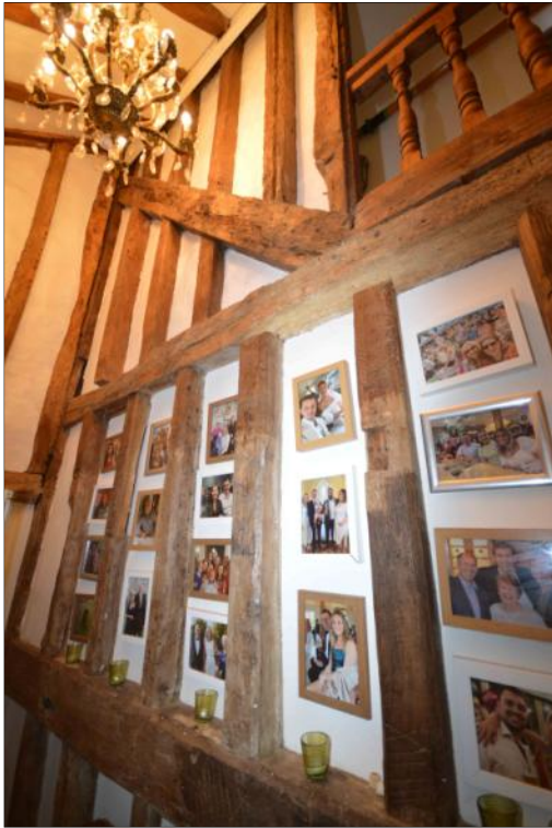
Plate 5: Details of the regular studs and straight raking shores in the rear wall of the main range, between it and its integral outshot
