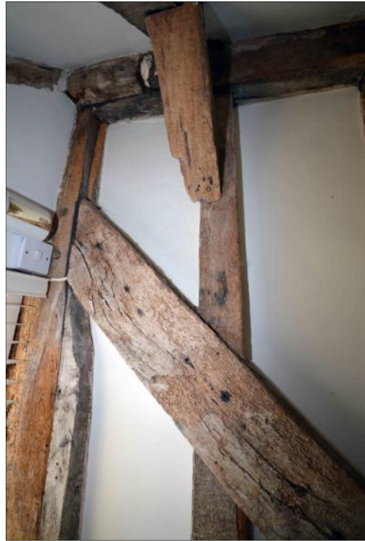
Plate 5: Details of the regular studs and straight raking shores in the rear wall of the main range, between it and its integral outshot
