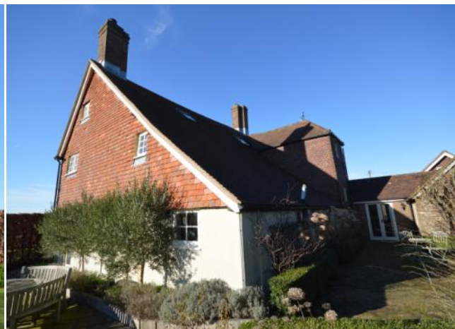
Plate 2: The south end showing the attics, rear outshot with catslide roof and integral stair turret
