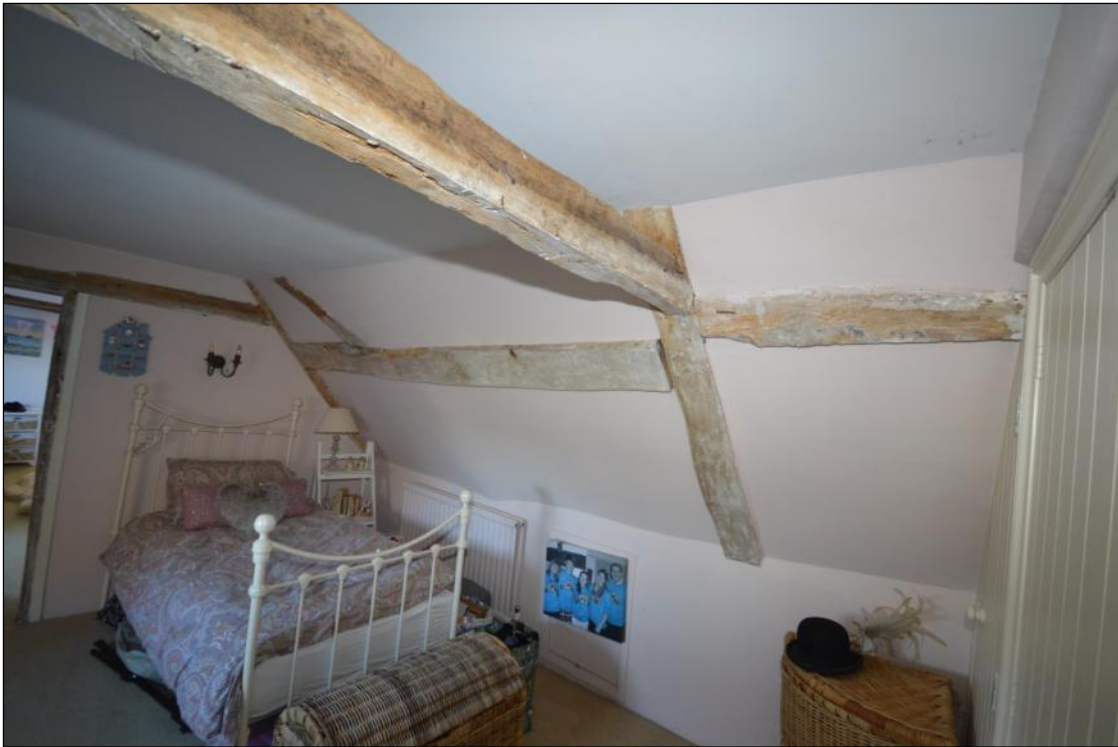
Plate 7: Butt-purlin roof structure
