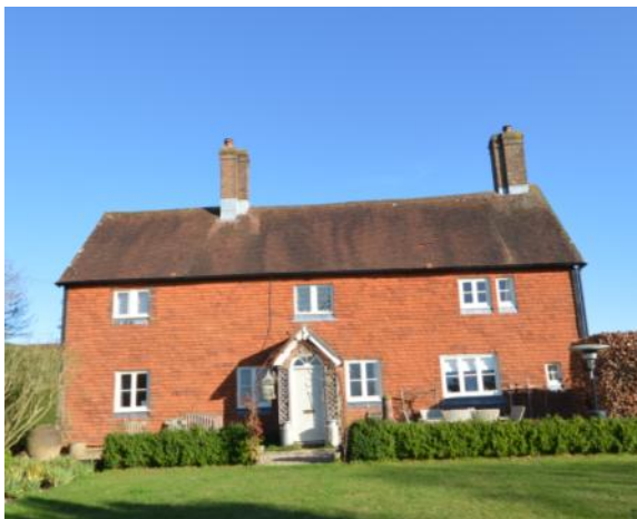
Plate 1: The west facing, principal elevation of Bishops Place
