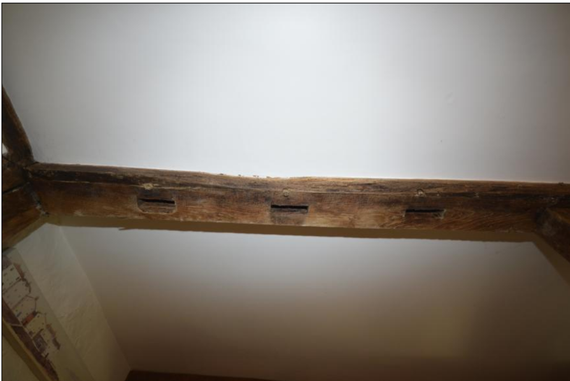
Plate 4: Detail of the soffit of the side girt between the main range and outshot at the south end of the house showing the mortises for regular studs
