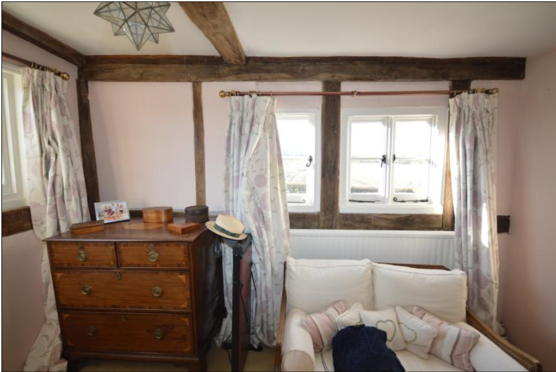
Plate 3: Small panel framing on the west elevation of the main range
