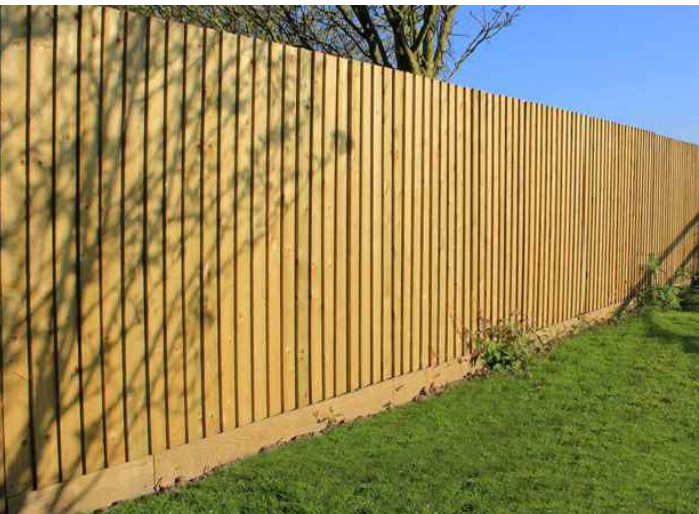
2.0m Close-boarded timber fencing with gravel board
