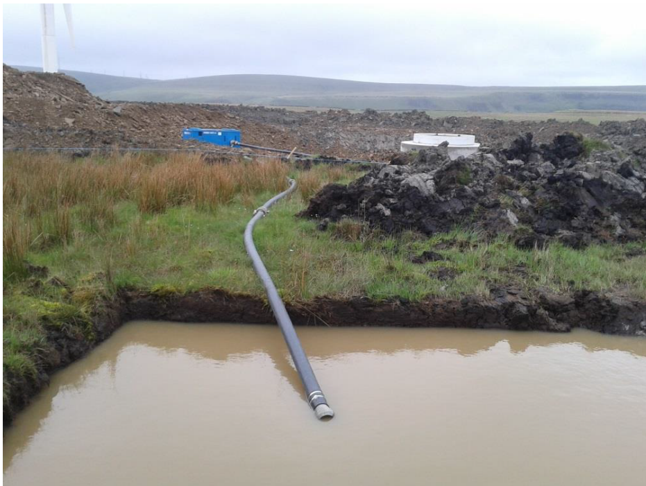
Figure 3: Typical 'Siltbuster' and settlement lagoon
