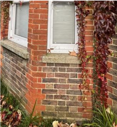
Existing brown multi-stock bricks with red brick detailing.
