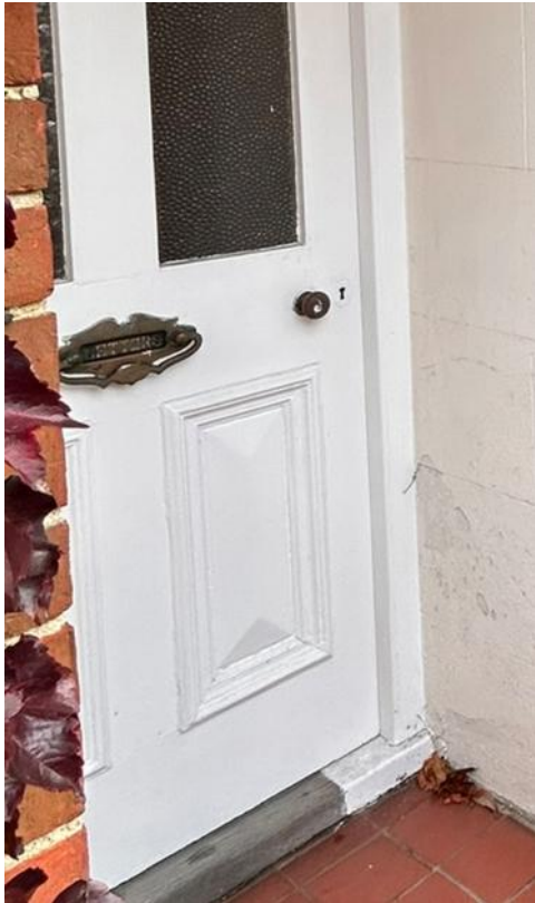
Existing door design to be replicated. Detail of plain glazed upper panels & raised bolelection mouldings to the lower panels.
