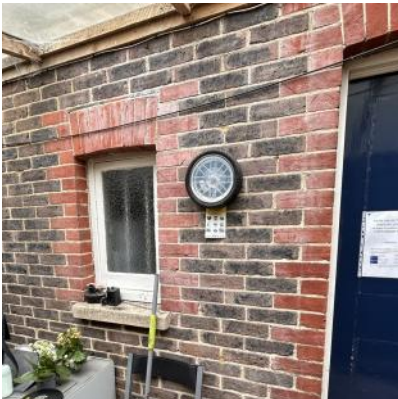
Existing plain red brick detailing around openings
