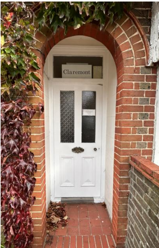
Existing door design to be replicated. Detail of plain glazed upper panels & raised bolelection mouldings to the lower panels.
