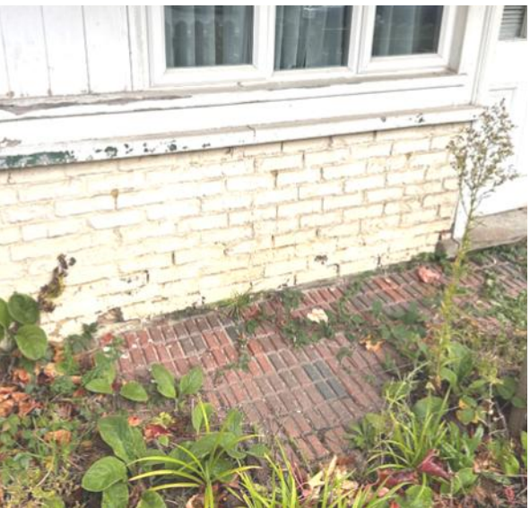
Shop front original brick paving
