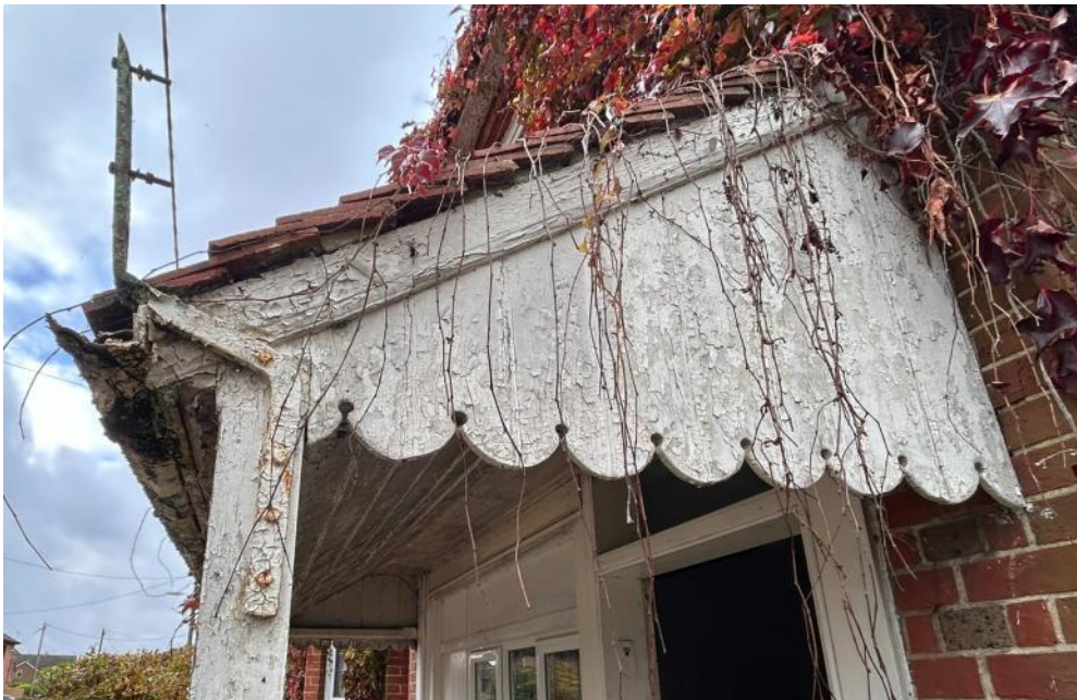
Shop canopy side panels
