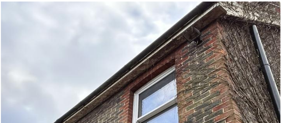
Existing roof eaves with closed soffit to be replicated. No visible eaves ventilation fixings.
