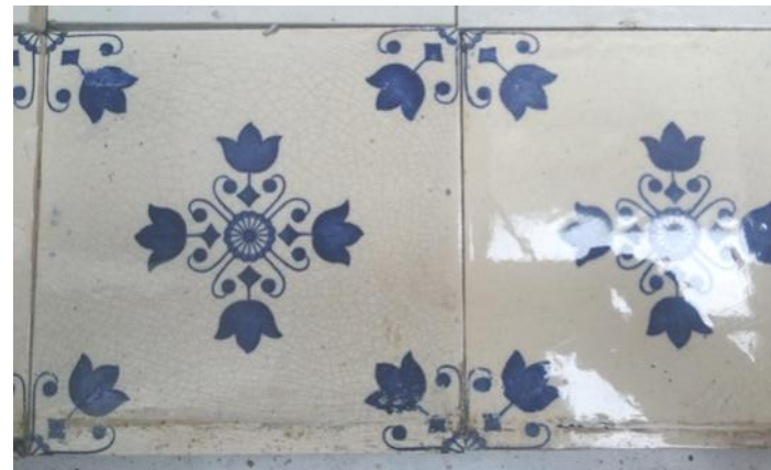
Original tiles to be reinstated
