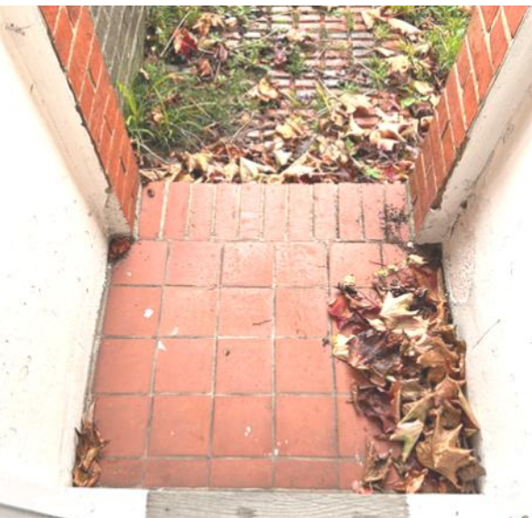
Front door existing quarry tiled entrance porch with brick path to front boundary
