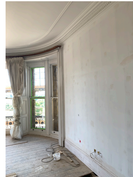
Example of cornicing and skirting retained
