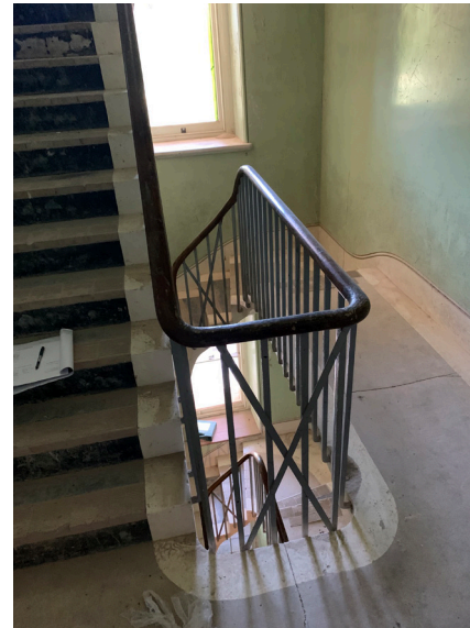
Example of existing stairwell balustrade retained
