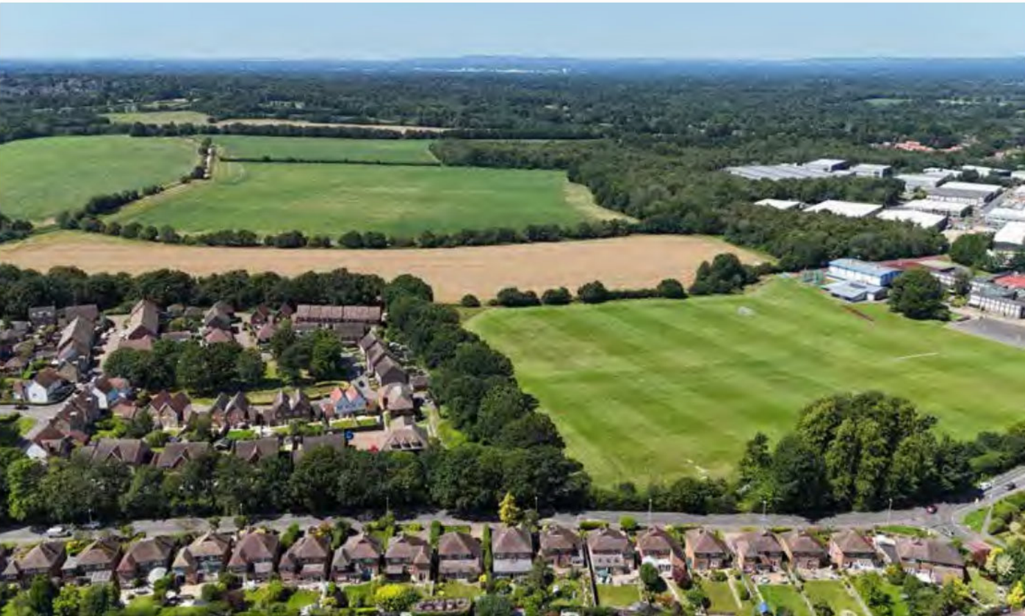
FIGURE 2.11: AERIAL PHOTOGRAPH OF THE SITE
