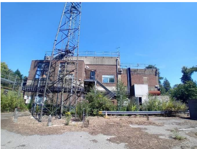
Plate 23: Rear of the of the EDF Energy building – location of WLS108.
