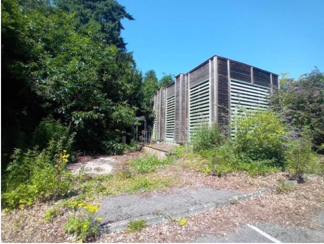
Plate 25: Air conditioning plant to the southwest of the EDF Energy building – location of WLS109.
