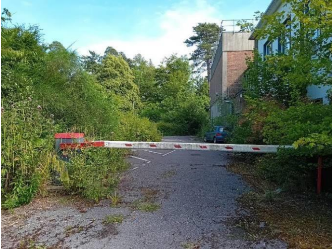
Plate 13: Access on the east of the site, leading to the rear of the EDF building.
