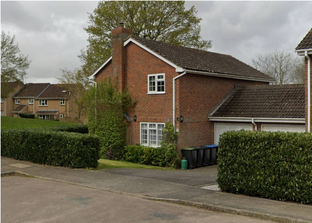
Image 1 – View from streetview of the garage and parking
