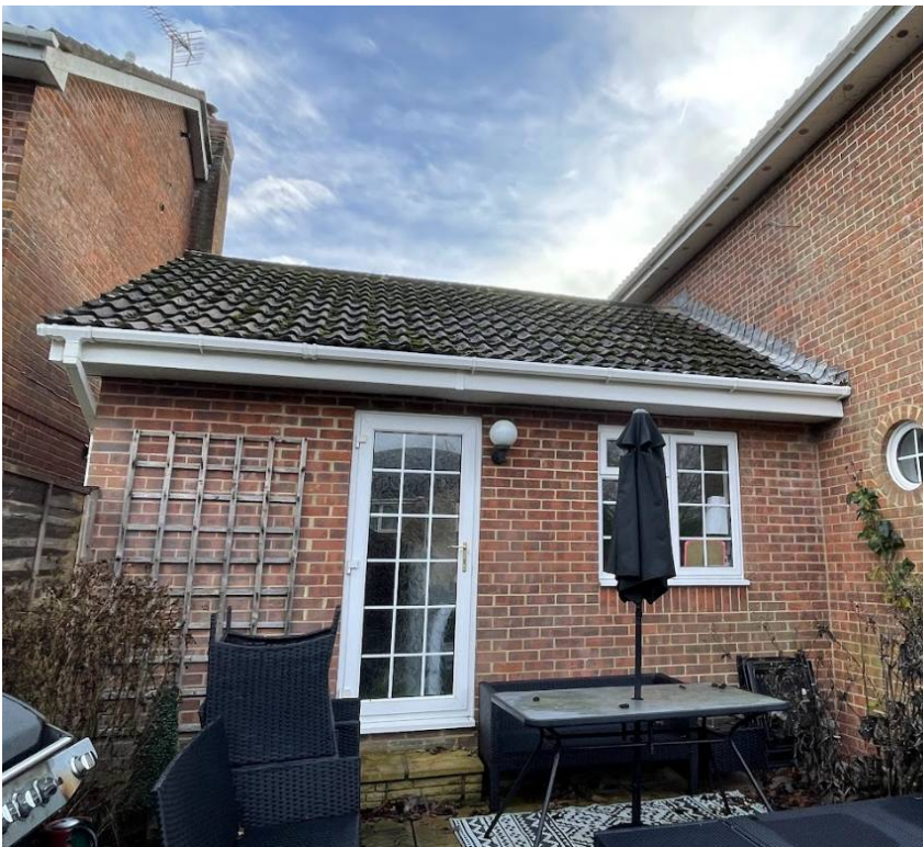
Photograph 2 – View of the rear of the existing garage
