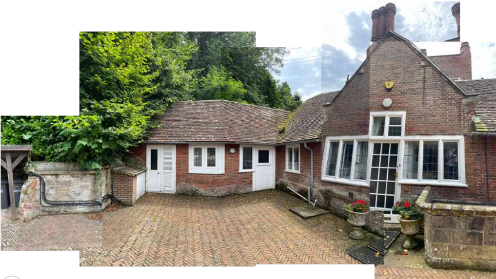
A1 External view of gym and utility to be removed/extended
