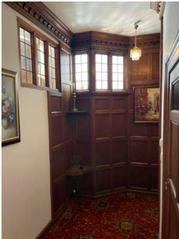
B1- New entrance door to be formed in area of panelling adjacent to HL window
