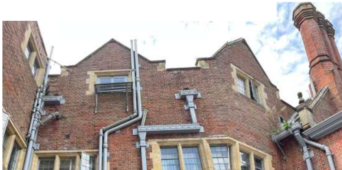
C2 - View of existing elevation from courtyard
