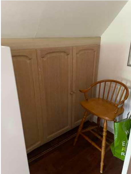
K Wall (right) to be removed
