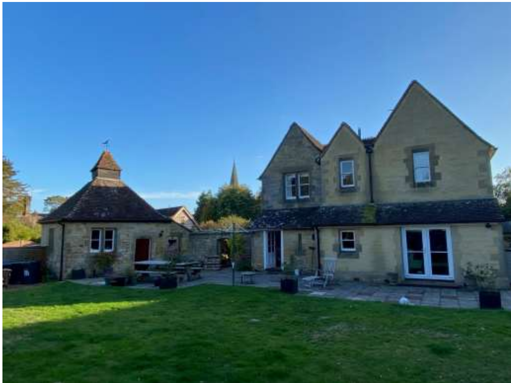
Figure 6: St John's Lodge viewed from the north. The 1984 extension is visible to the right (textured render finishes) and bothy outbuilding to left. The spire of All Saint's Parish Church is in the distance.
