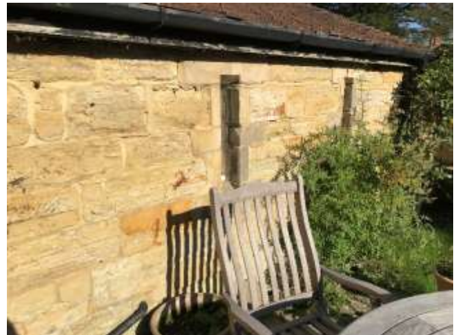
Figure 20: Examples of poor quality cementitious mortar pointing and smeared render repairs to the main dwelling, link wall and former Bell Tower (bothy) resulting in the rounding of ashlar stonework.
