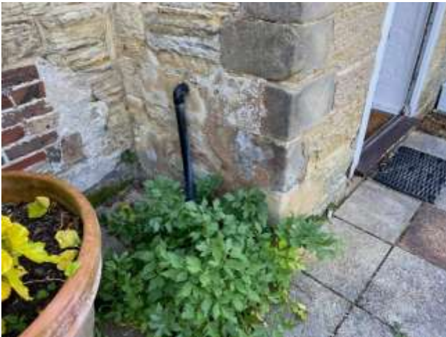
Figure 20: Examples of poor quality cementitious mortar pointing and smeared render repairs to the main dwelling, link wall and former Bell Tower (bothy) resulting in the rounding of ashlar stonework.
