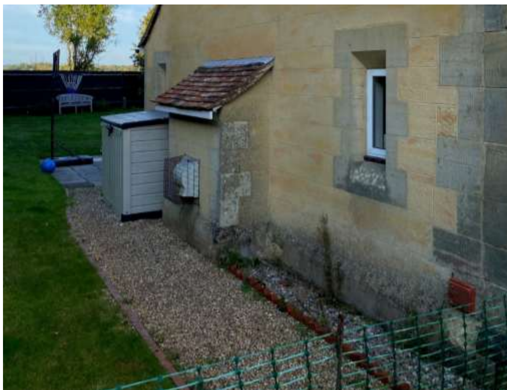
Figure 28: Detail of contrived 'tooled stone' ashlar finishes to 1984 extension
