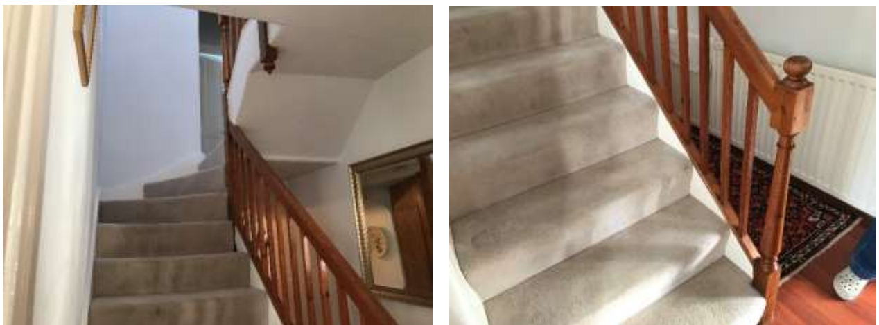
Figure 24: The half turn winder staircase.
