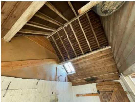
Eastern section of the Former Stable roof
