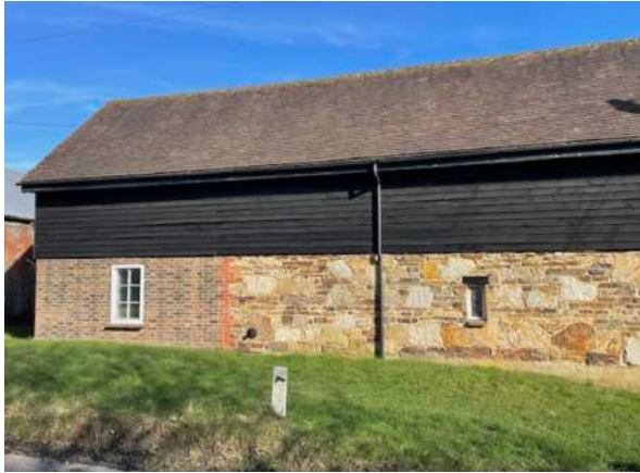
Annex Area 1a External western wall
