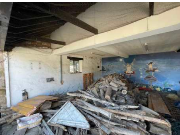
Annex Internal Garage
