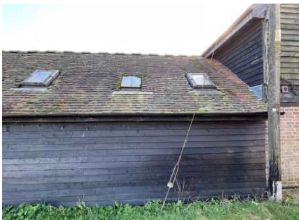
Former Stable- Area 1b external wall
