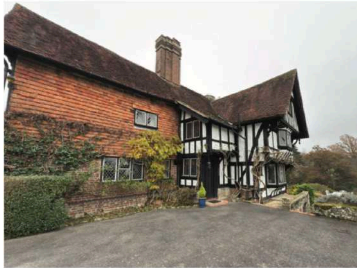
C17th range (western wing & southern gable)
