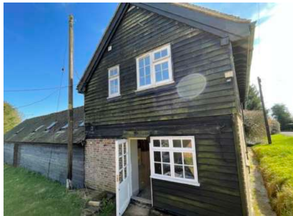
Annex Area 1a End termination northern wall
