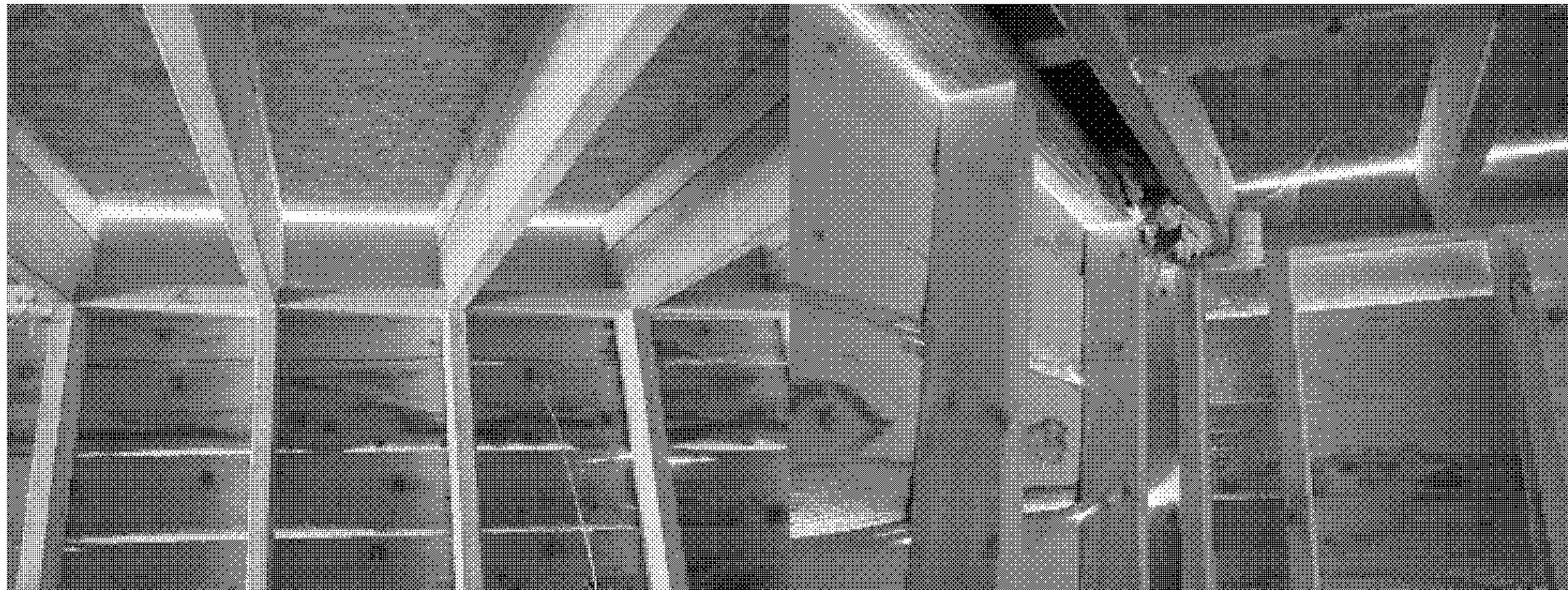
Photograph No: 5 – Gaps between wooden slats within B01.
