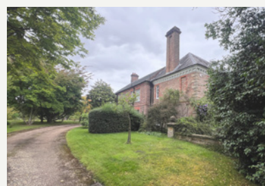
5. DRIVE ALONG WEST ELEVATION
