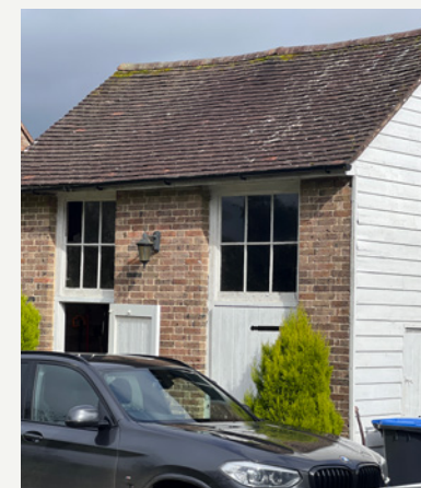
TOOL SHED ENTRANCES
