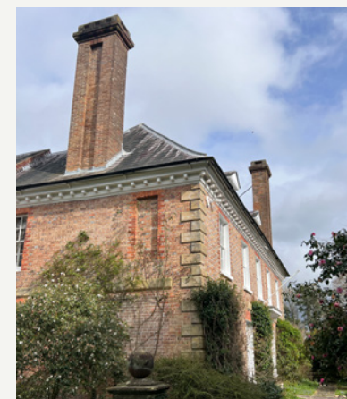
SOUTH-WEST ELEVATION CORNER
