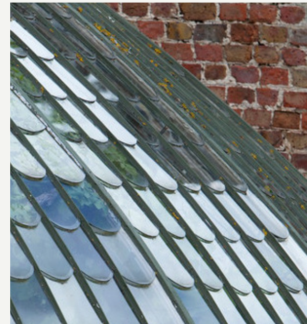
'PAXTON' GLASS AND SHAPED PANES
