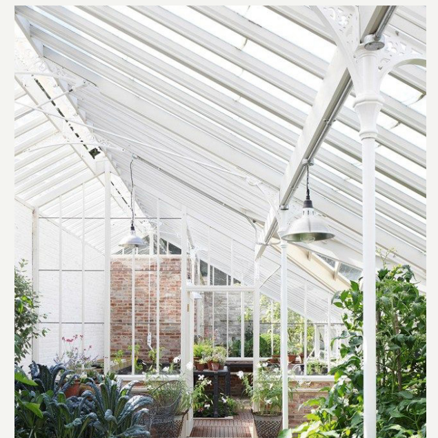
LEAN-TO FORM WITH SHAPED METALWORK
