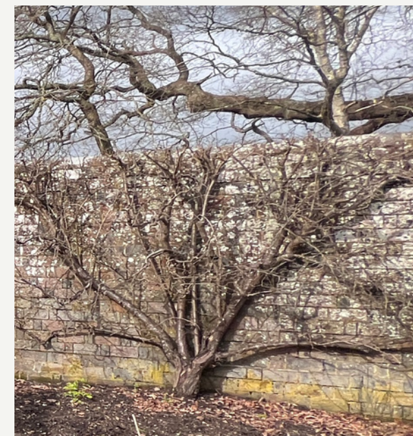
EXISTING BRICK WALL
