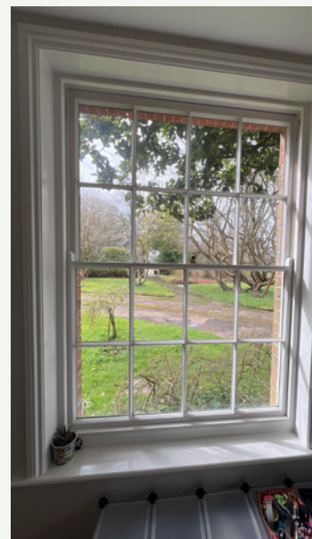
L00 WEST FACING FROM KITCHEN
