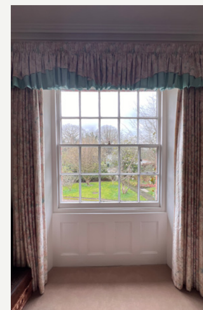
L01 WEST FACING FROM BEDROOM
