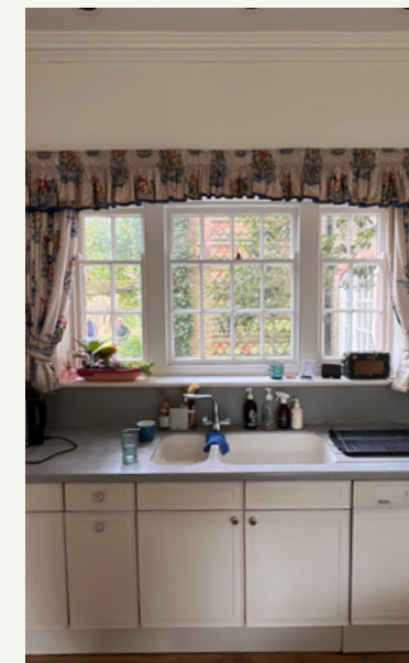
L00 EAST FACING WINDOW TO COURT
