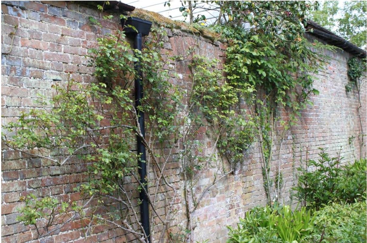
Figure 53: Plate 18 - Blocked up door on the west wall of the formal garden
