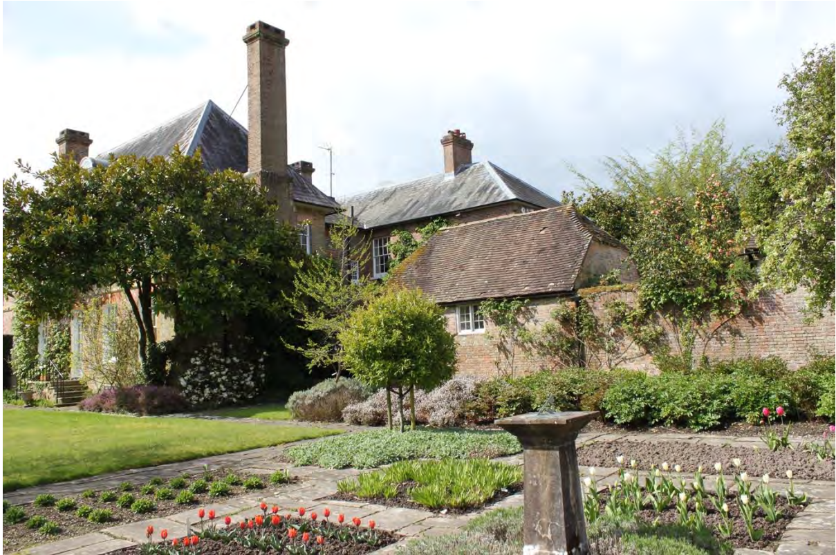
Figure 52: Plate 17 - View of the west wall adjoining the dairy from the east looking southwest
