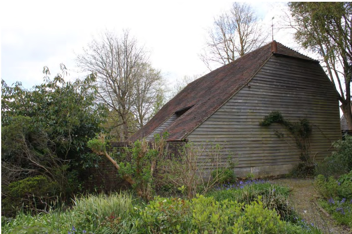
Figure 61: Plate 26 - View of the south elevation of the barn from within the garden looking northeast
