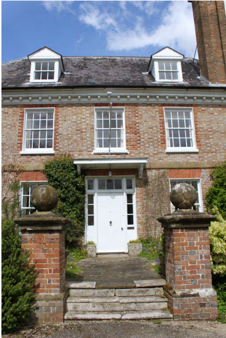
Figure 42: Plate 7 - View of the central section of the south elevation looking north
