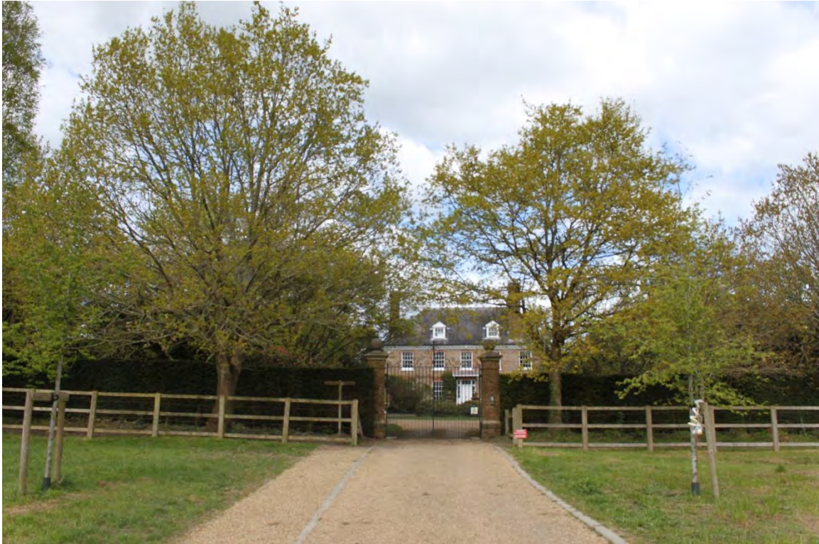
Figure 38: Plate 3 - View of the south elevation from the top of the approach looking north.
