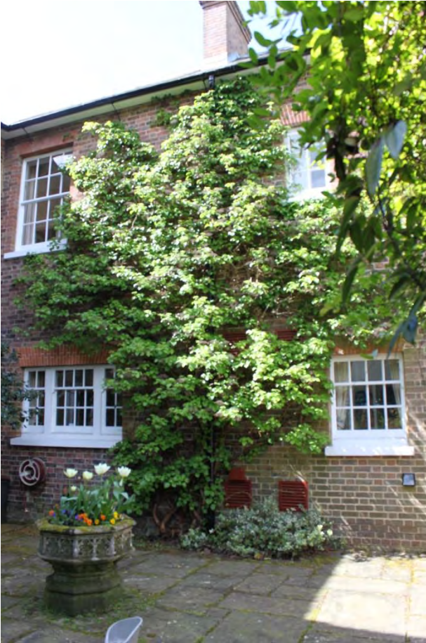
Figure 84: Plate 49 - Rear east elevation looking west
