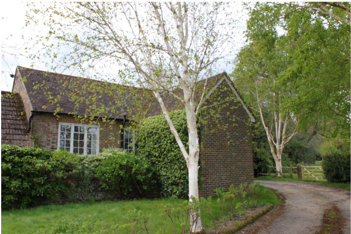
Figure 73: Plate 38 - Rear of the cottage north elevation looking southwest
