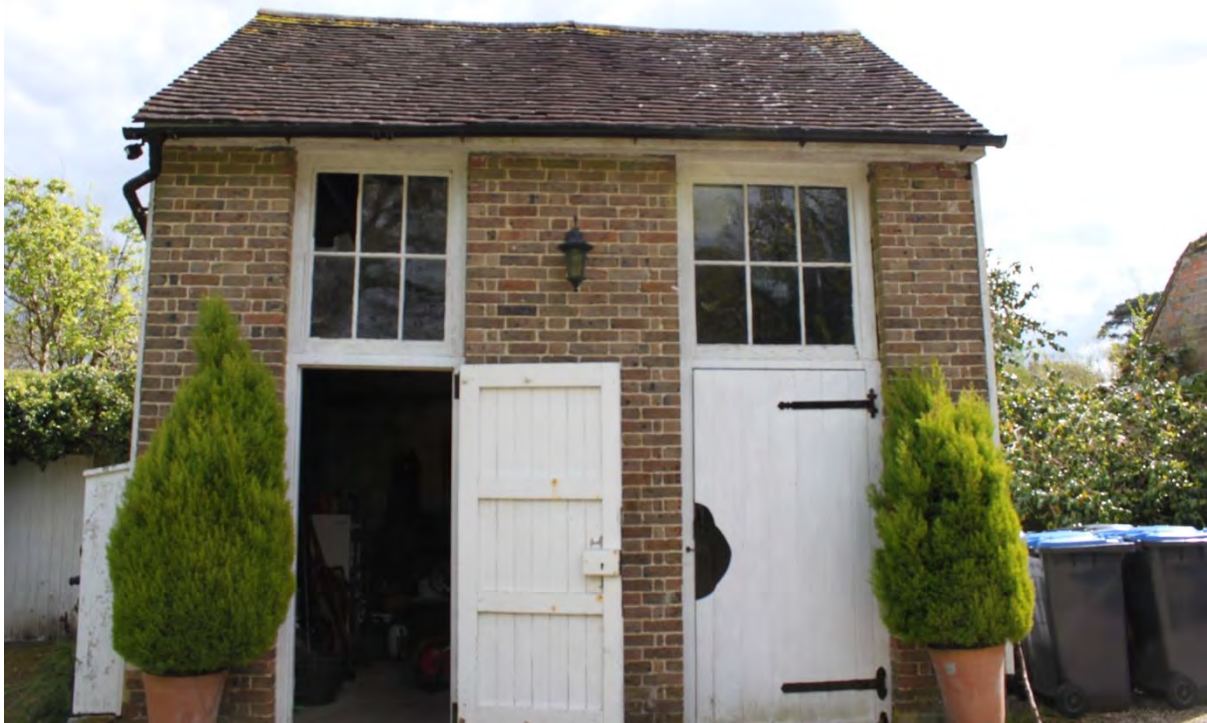
Figure 76: Plate 41 - View of the west elevation of the tool shed from the west looking east
