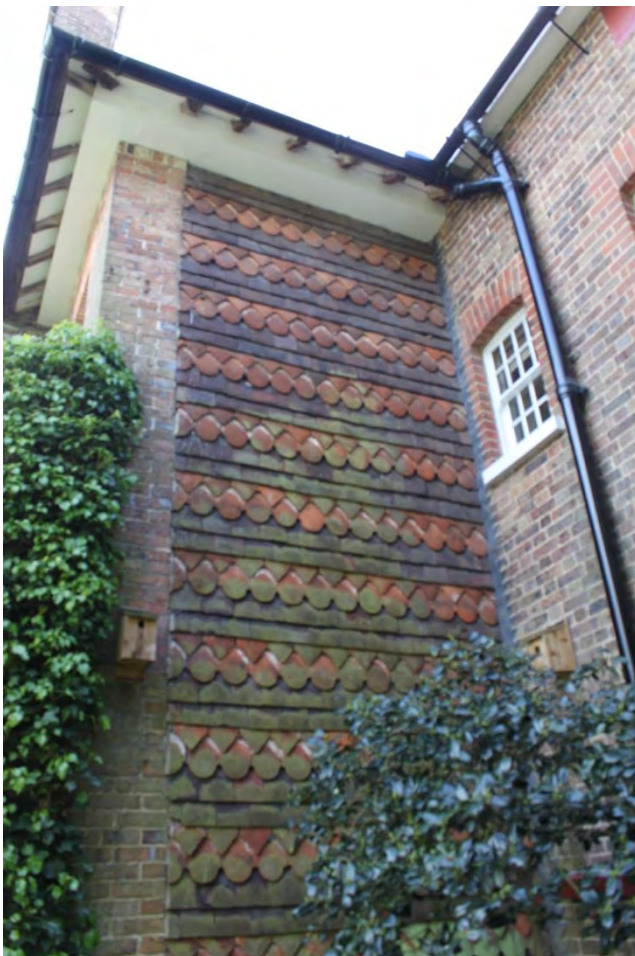
Figure 81: Plate 46 - Rear west courtyard elevation looking southeast
