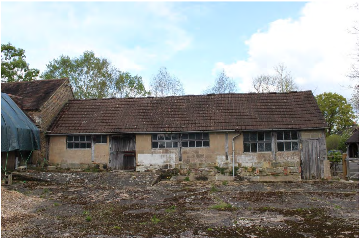
Figure 67: Plate 32 - View of the stables from the south looking north
