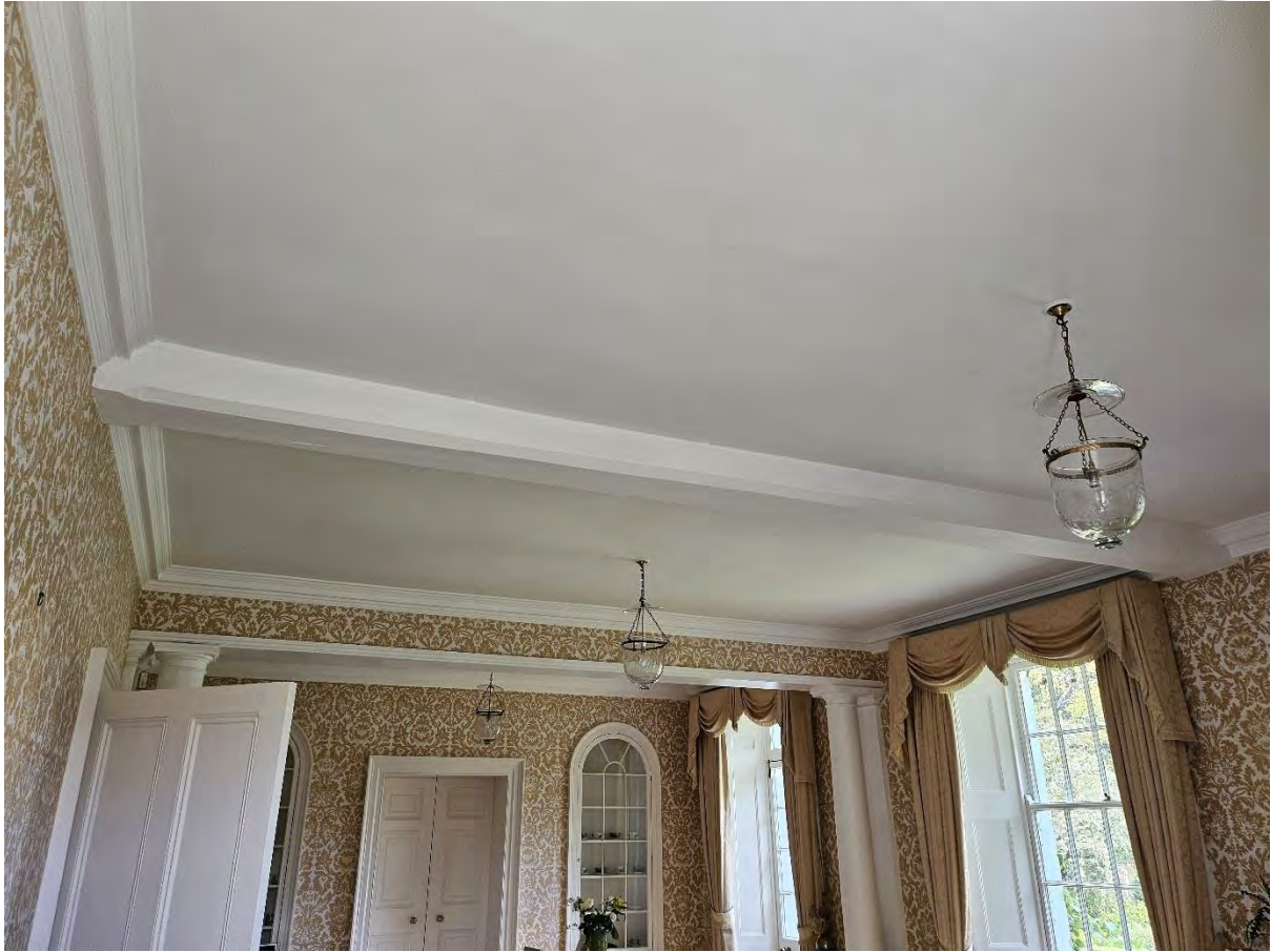
Figure 94: Plate 59 - Sitting room – view to the timber chamfered beam
