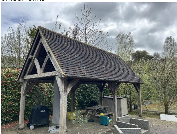
S1 – Outside dining shelter
