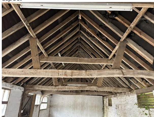
B6 Stable – internal roof structure
