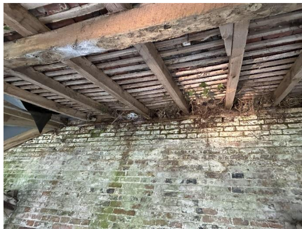
B8 Byre – internal roof structure with evidence of nesting birds
