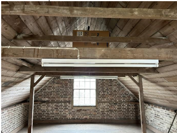
B4 Garage – internal roof structure
