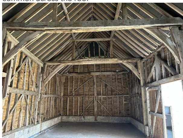
B9 Barn – internal roof structure
