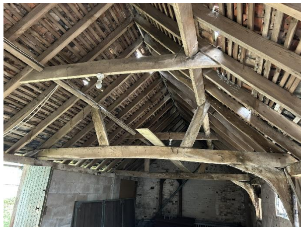
B7 Cowshed – internal roof structure
