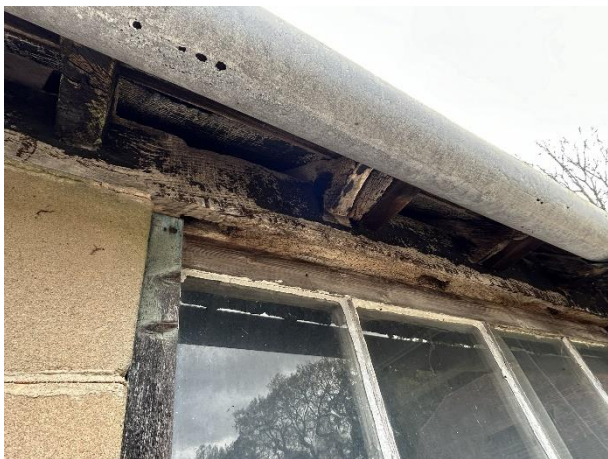
B6 Stable – exposed, open eaves at southern aspect
