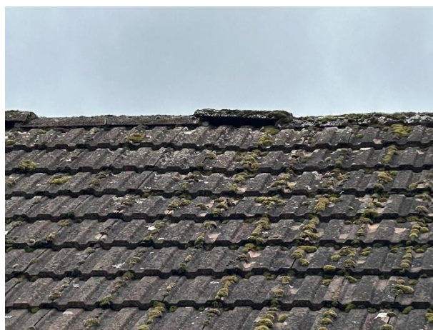
B6 Stable – vented ridge tiles and tightly fitted concrete tiles
