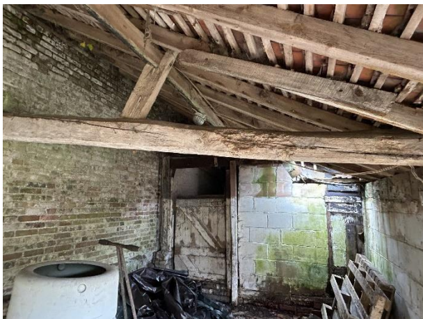
B8 Byre – internal roof structure with access door into B7
