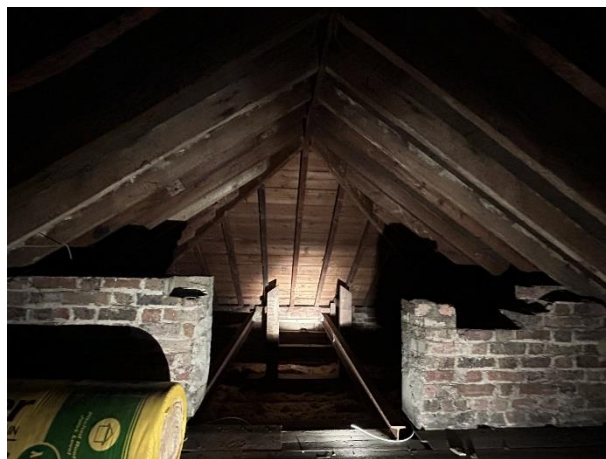
B1 Main House – Void V2
