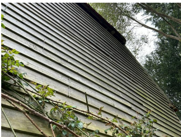
B9 Barn – example of lifted timber panels on southern aspect
