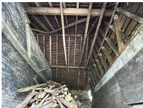
B3 Log shed – internal roof structure with timber panelled external walls.
