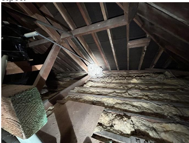
B1 Main House – Void V1
