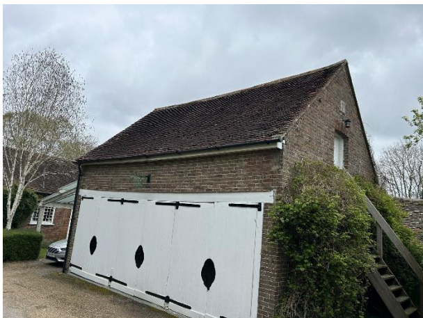
B4 Garage – south-west aspect
