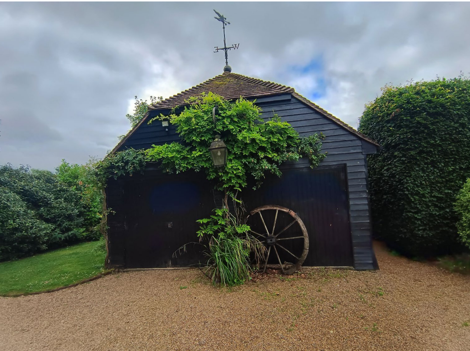
North Elevation of Garage
