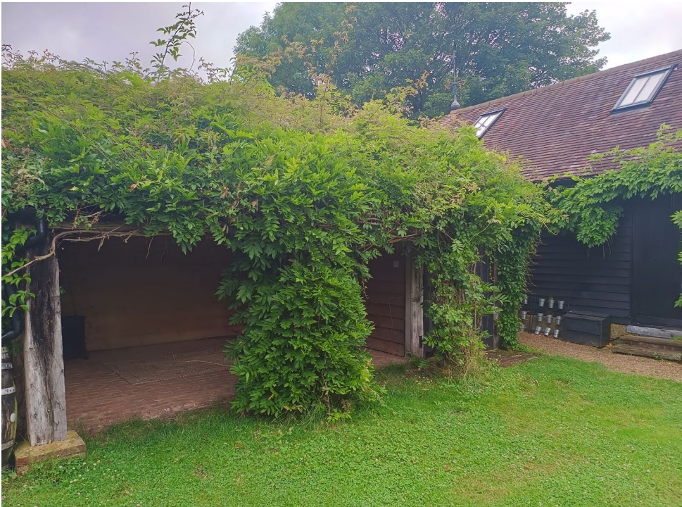
South Elevation of Loggia
