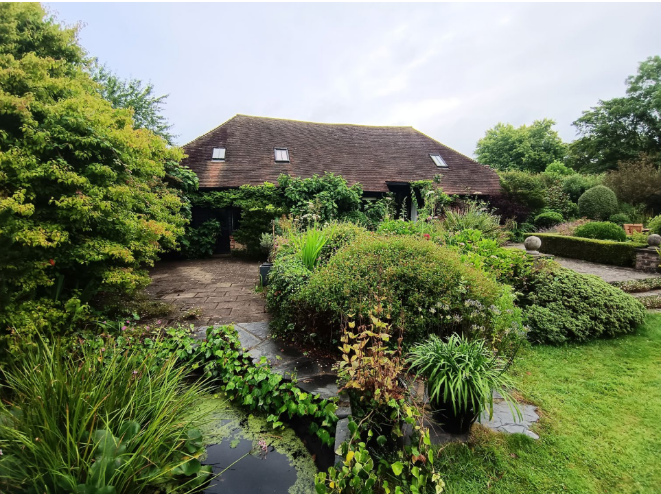
South Elevation of Main Barn
