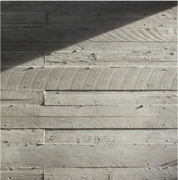
Board marked concrete
