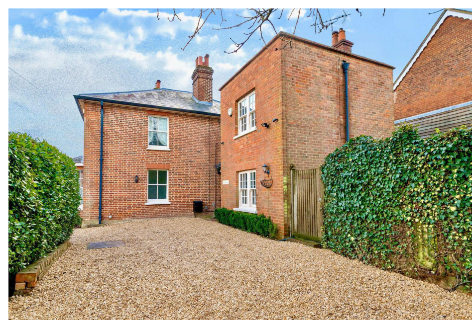
Sample Gravel Drive
