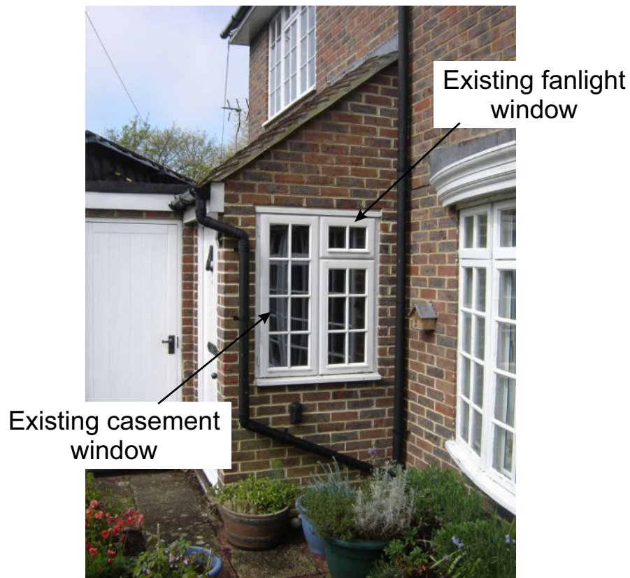
Existing arrangement of casement and rectangular fanlight windows
