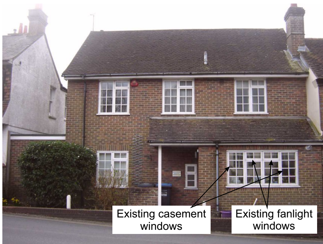
Existing arrangement of casement and rectangular fanlight windows
