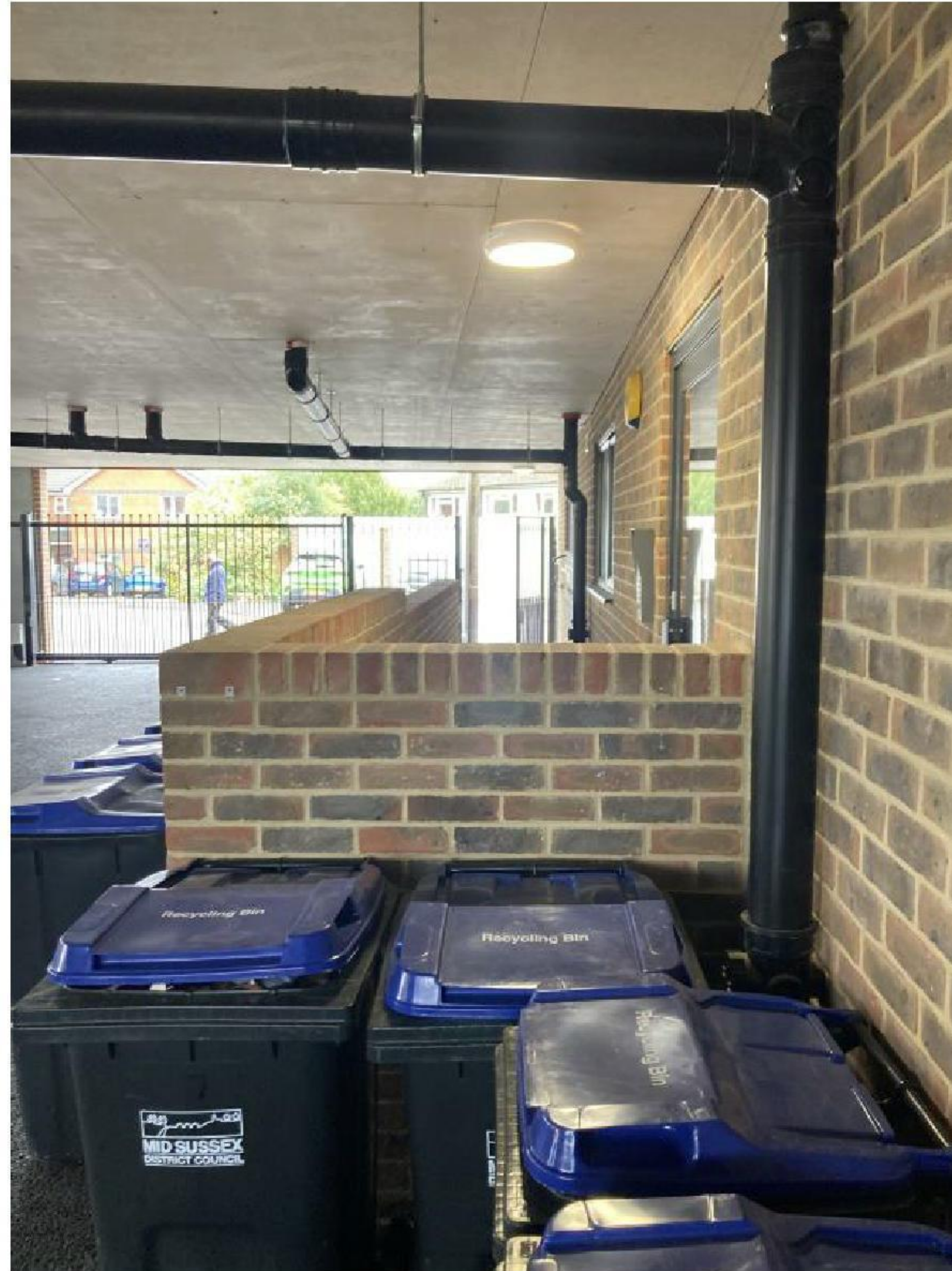
Low wall and bins
