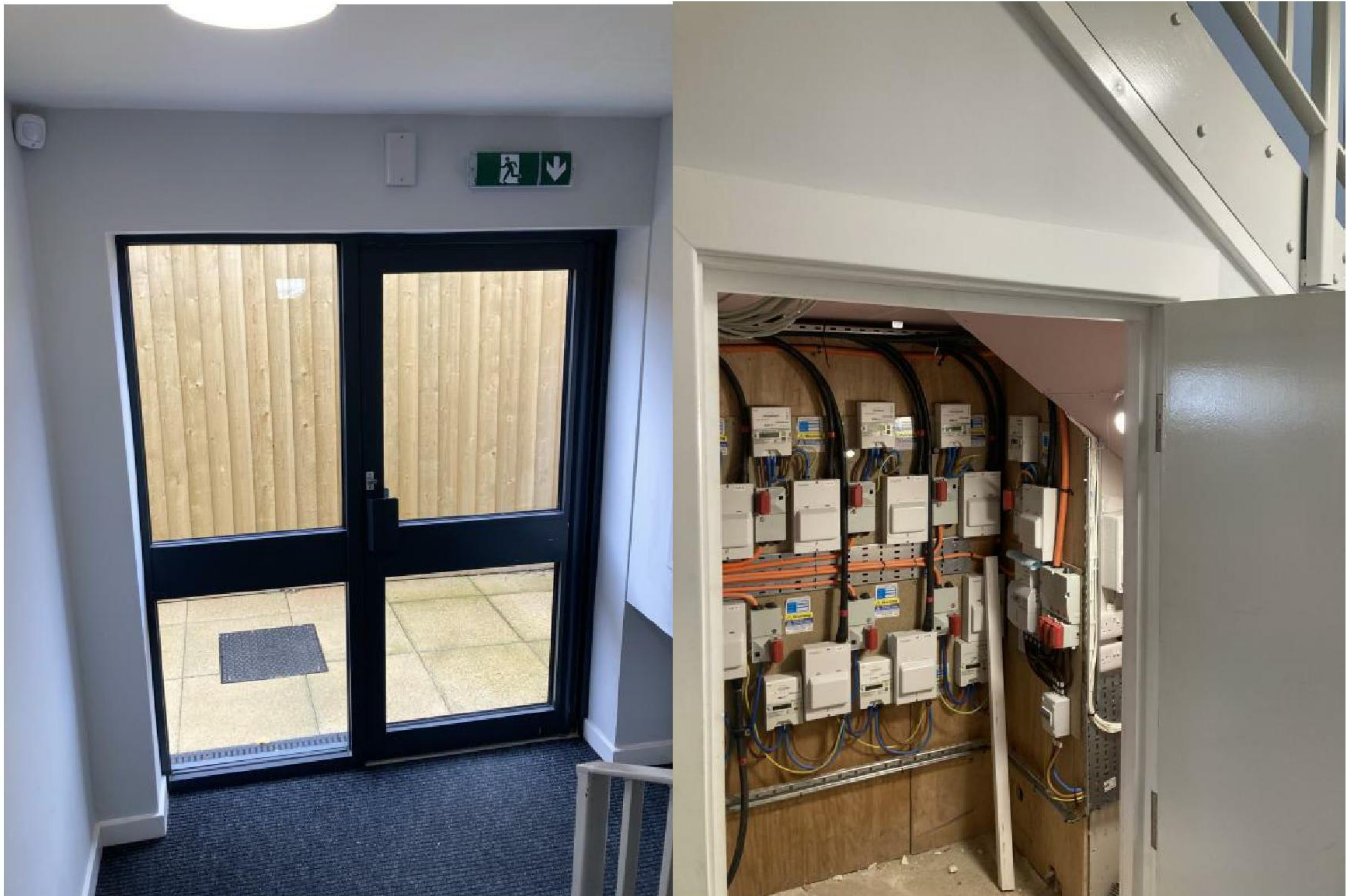
The opaque glass is now our back door and access to the bin and bike stores, with the electrical cupboard in place of the hallway to a dedicated entrance
