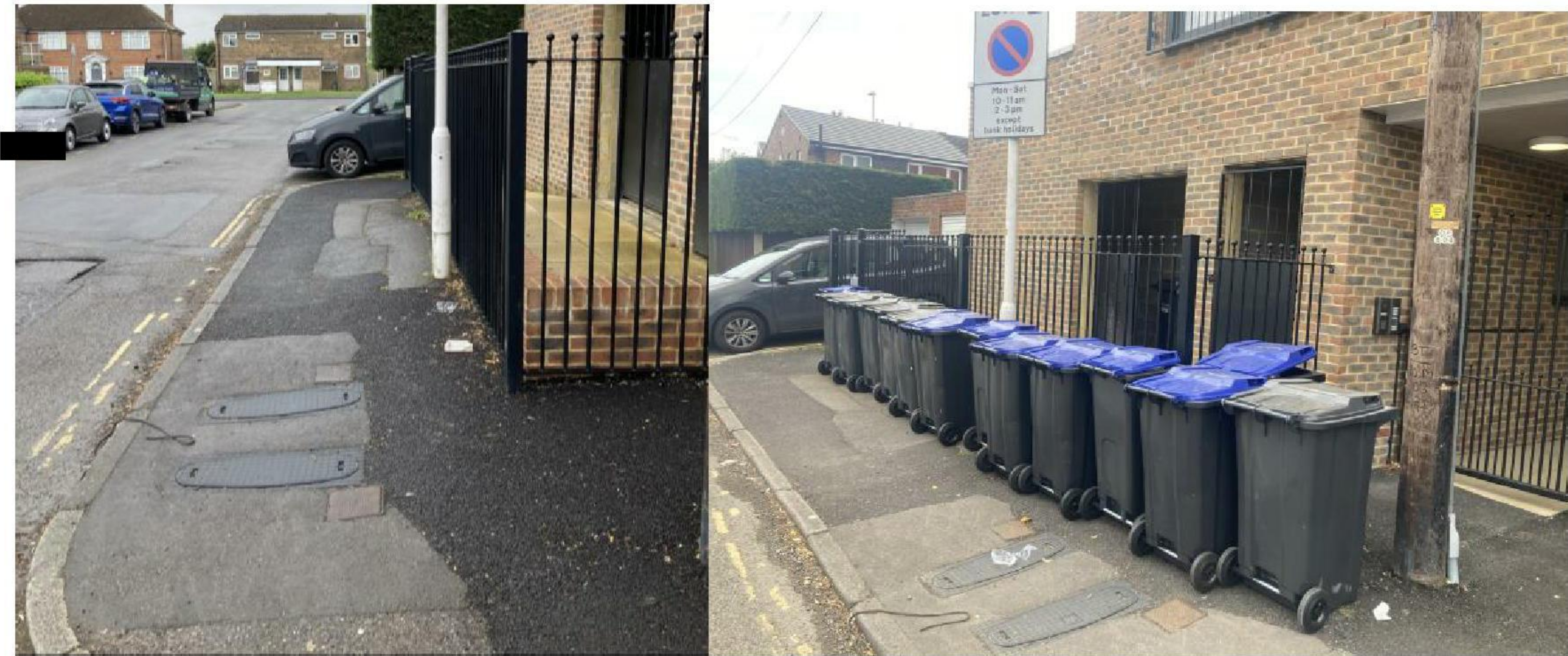
18 bins at a time are brought out here due to deviations from approved planning; bin day (not all 18 bins)
