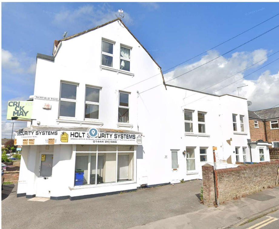
External view of the building (side)
