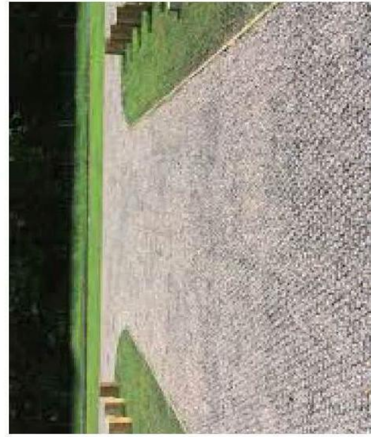
P5 - Ground reinforcement grid system with gravel fill Supplier: Geosynthetics Ltd or similar Type: Golpla Gravel: Buff in line with grid suppliers recommendations
