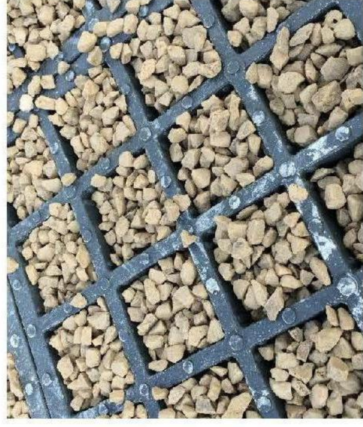
P3 - Ground reinforced grid system with gravel fill Supplier: Geosynthetics Ltd or similar Type: TTE (suitable for HGVs) Gravel: Buff in line with grid suppliers recommendations
