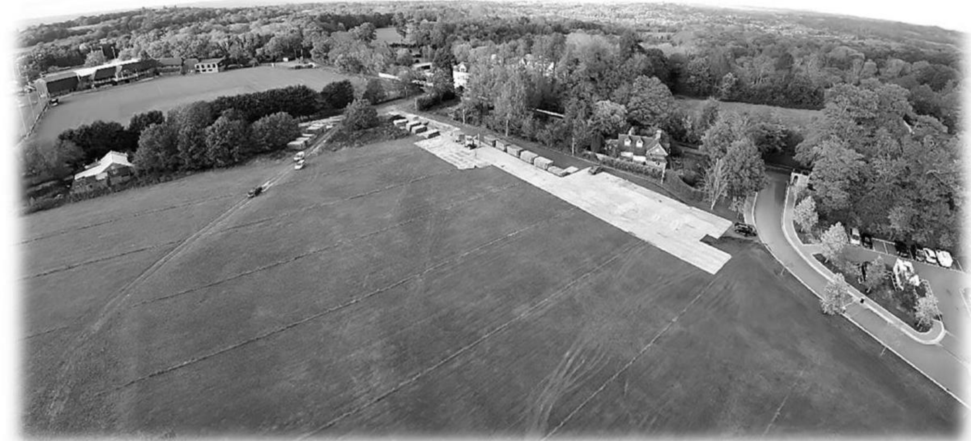
Image 16. Temporary Carpark plastic cover being installed. This area is similar to the proposed permanent parking in our design.
