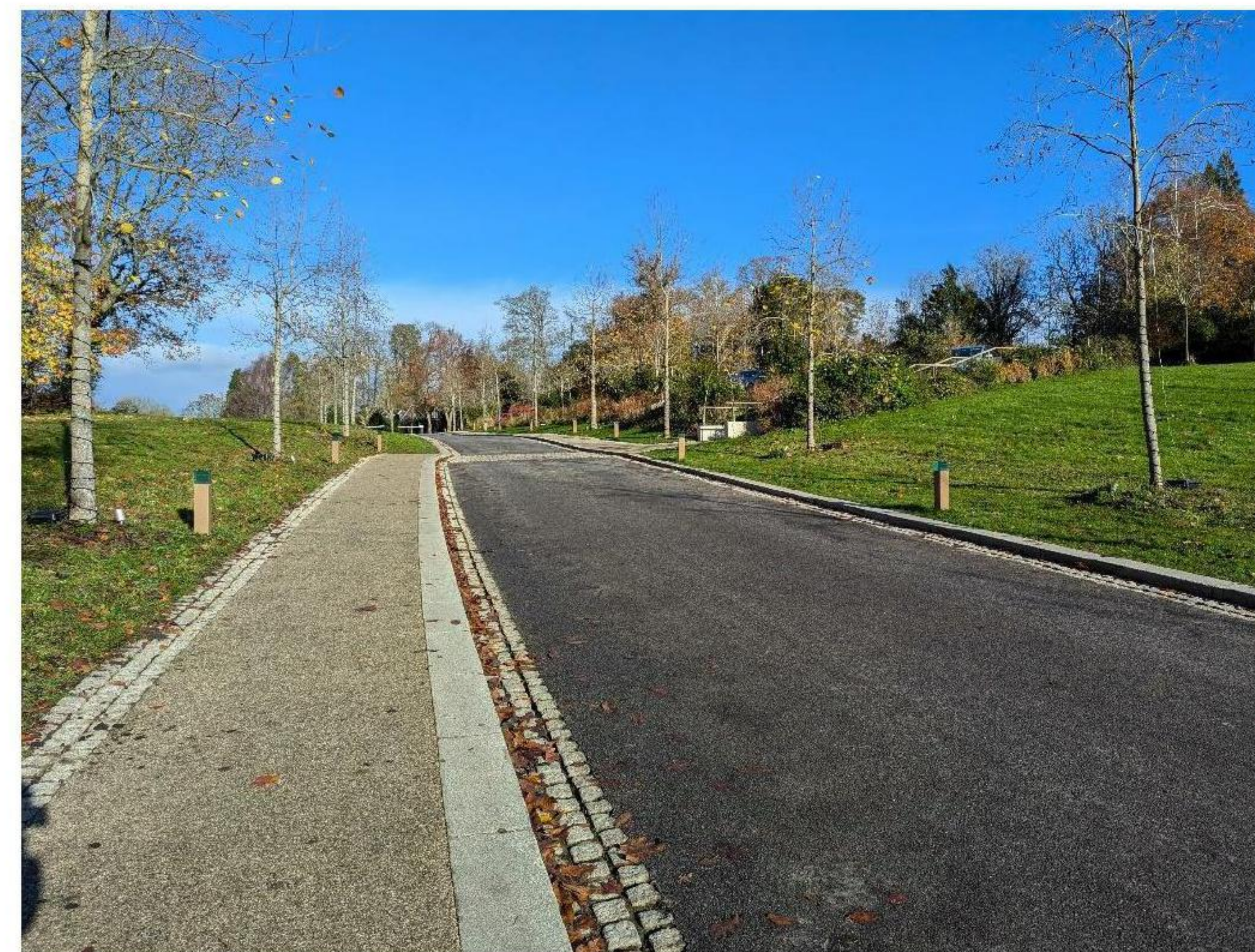
Existing footpath and road treatment at Saint Hill Manor
